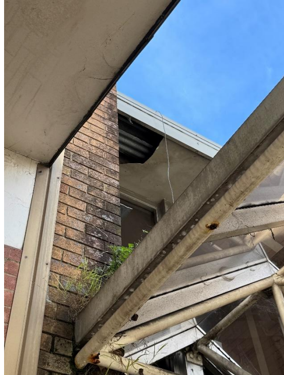
Figure 13: Opening under eave at 255-259 Pacific Highway.
