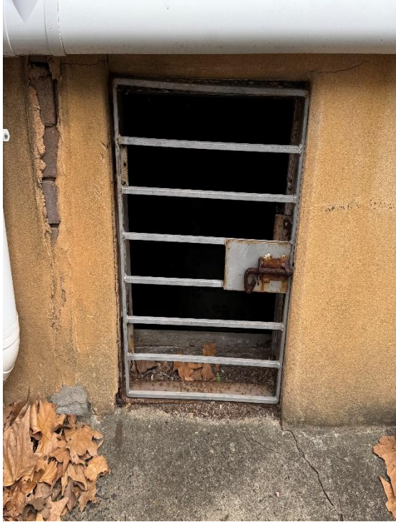
Figure 12: Potential entry point into underground space at rear of 253 Pacific Highway.
