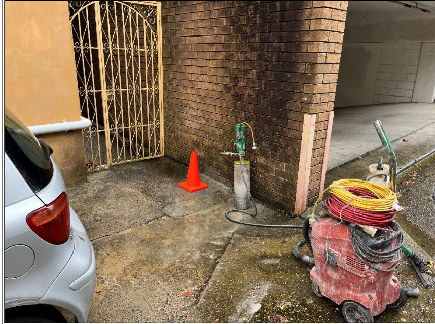
PHOTO 2: 253 PACIFIC HIGHWAY BH10 LOCATION, FACING NORTHWEST
