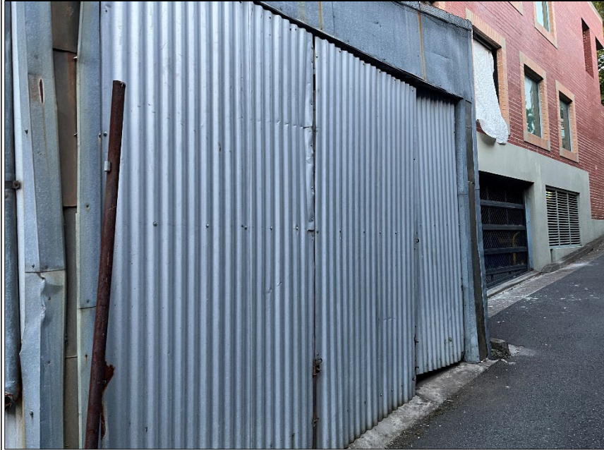
PHOTO 6: 265 PACIFIC HIGHWAY REAR ENTRY, FACING NORTHWEST
