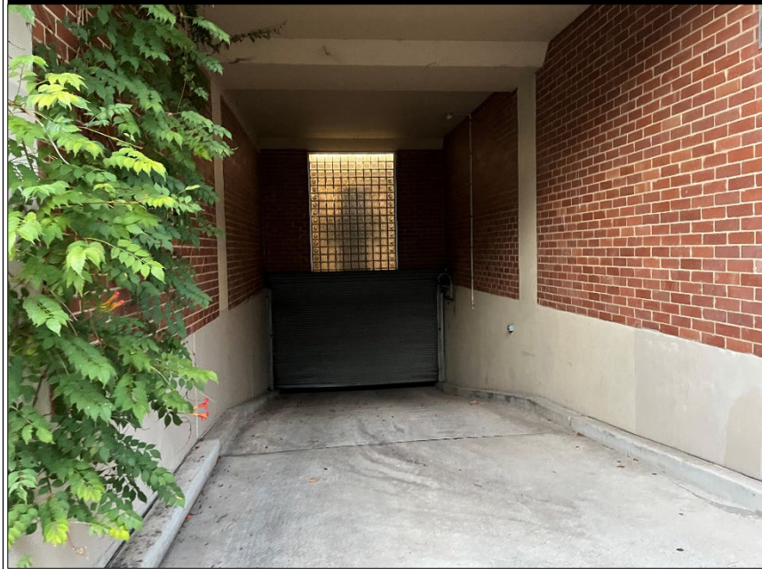
PHOTO 4: 261 PACIFIC HIGHWAY, FACING WEST
