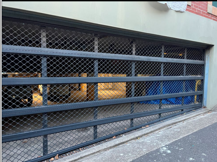
PHOTO 8: 267 PACIFIC HIGHWAY GARAGE, FACING WEST
