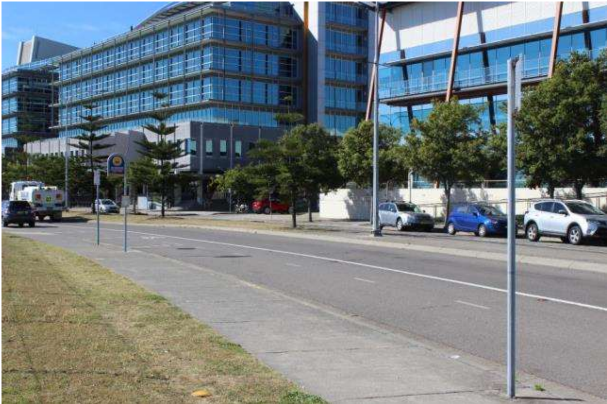
Photograph 7 – Existing bus stops immediately east of site.
