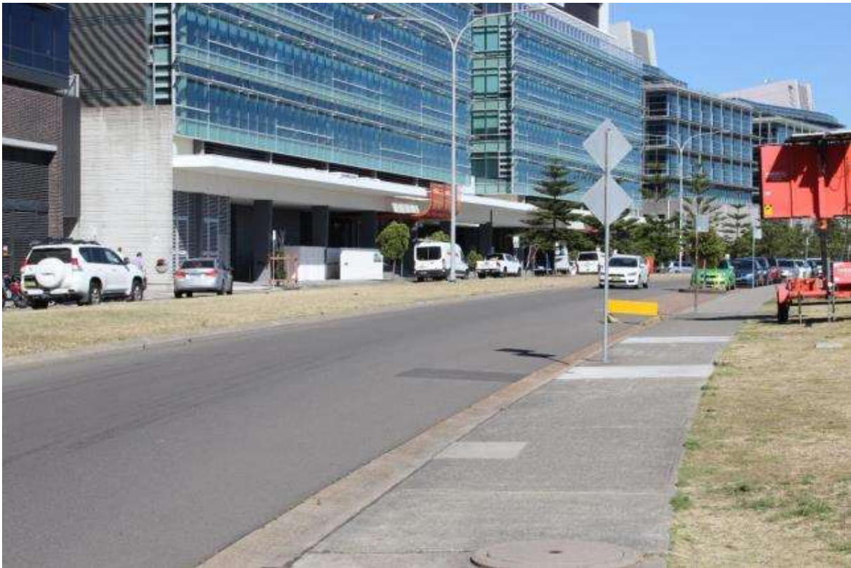
Photograph 10 – Pedestrian footpath – Honeysuckle Drive.
