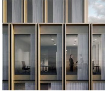
1. Metal cladding curtain wall facade in bronze colour.
