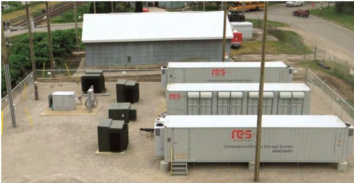
c) Example of energy storage (Lithium-ion batteries in containers)
