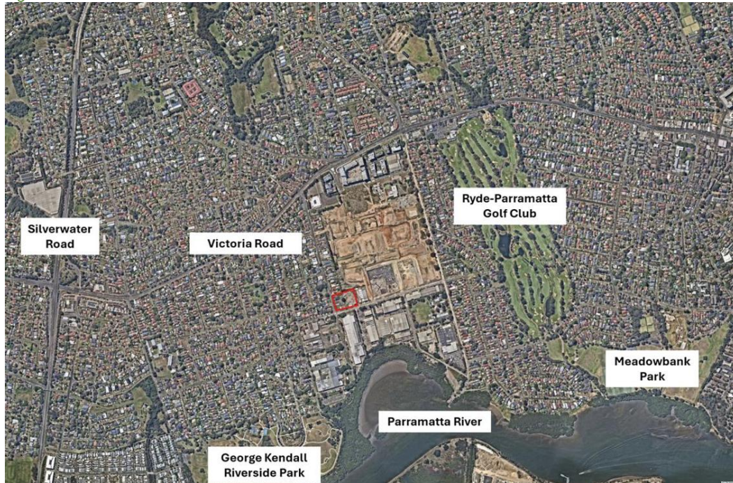
Figure 1: Site Location with site outlined red
