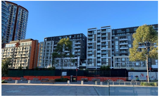
Stage 3 and 20-26 Ebswroth Street to the north east of the site
