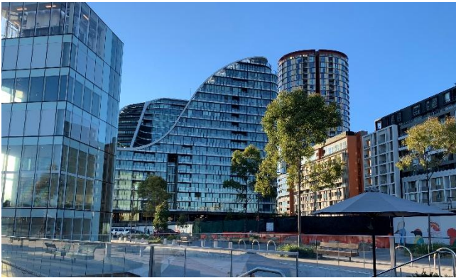
Stage 3, 'Infinity' and 'Ovo' developments to the north and north west of the site
