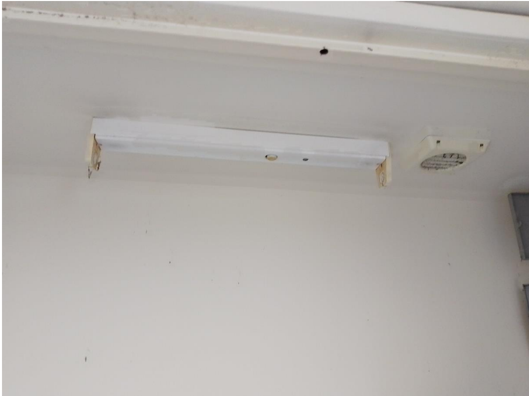
Photo 5: East wing, Garbage room, ceiling, fluorescent lighting fixtures, nil PCB (suspected).
