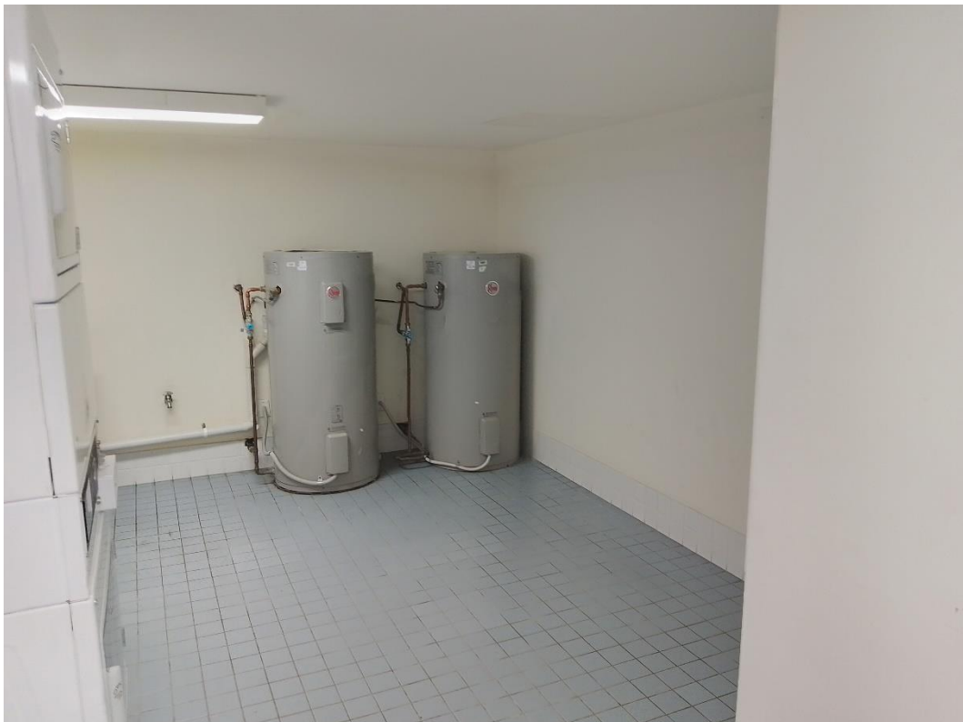
Photo 4: East wing, Common laundry 1, hot water units, internal insulation, SMF (suspected).
