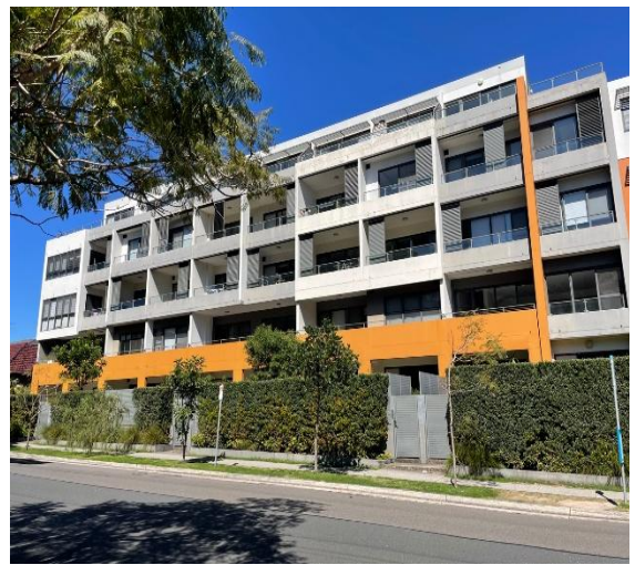
Figure 13 Opposite apartment building at 32 Barker Street
