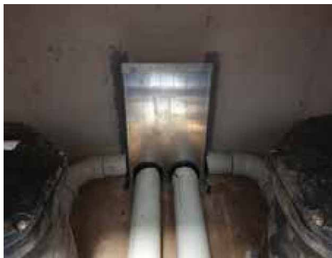
Figure 3 - Typical Outlet Weir Wall
