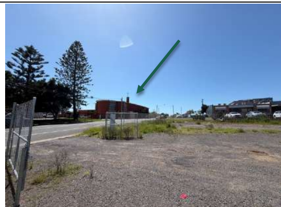
Looking from within the site toward the Heritage Item in a north easterly direction. The green arrow points toward Heritage Item Our Lady of the Rosary Catholic Church.
