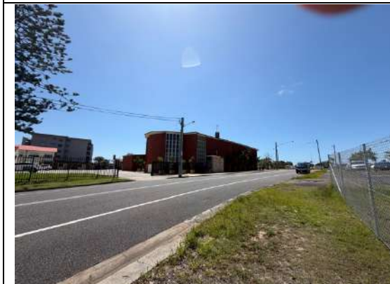
Looking from Ashton Avenue toward the rear of the Heritage Item 239-243 The Entrance Road, The Entrance in a north easterly direction.
