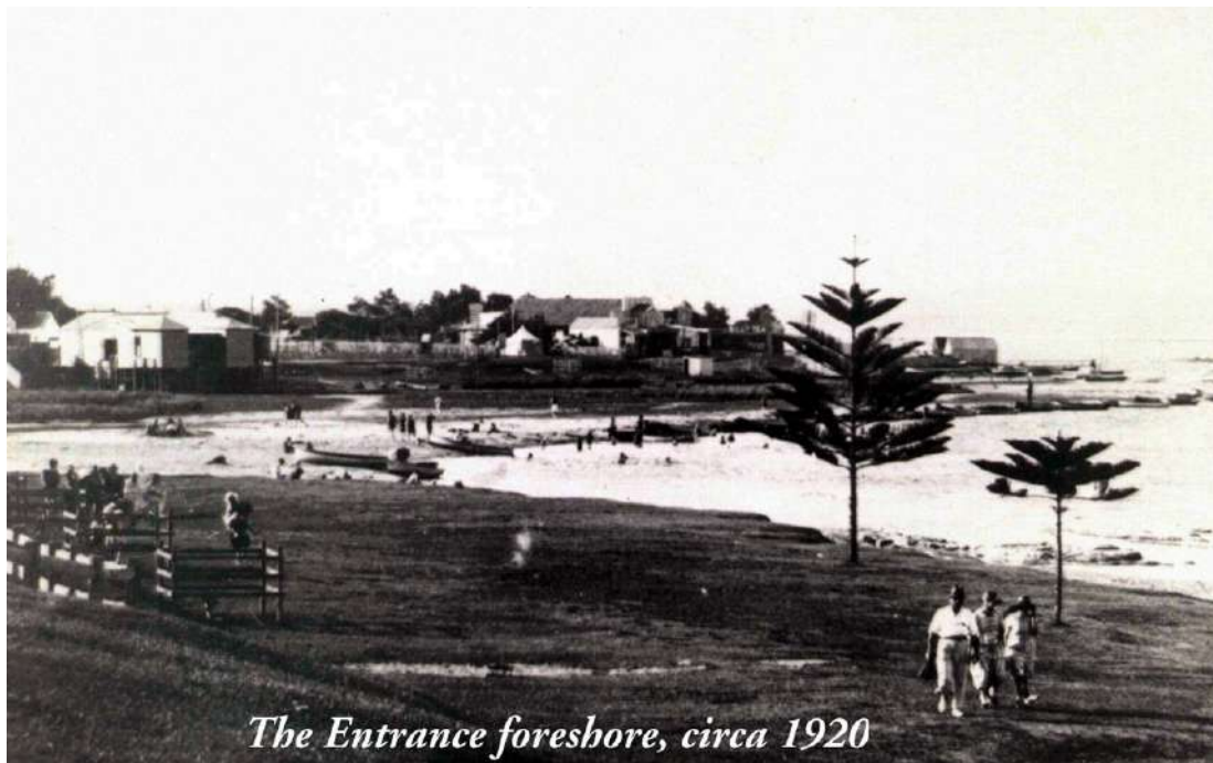
Figure 3 The Entrance Foreshore, The Entrance, NSW, c.1920.
