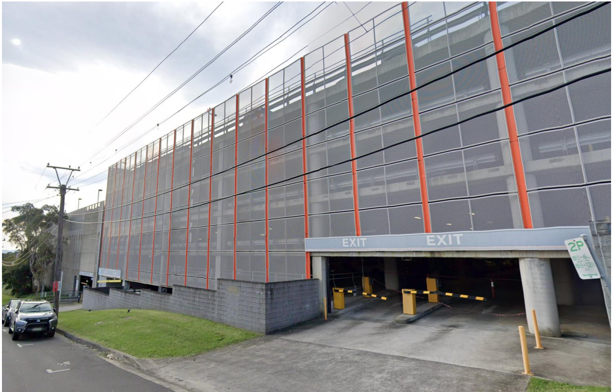
Figure 22 Wollongong Public Hospital carpark, as viewed from Dudley Street.
