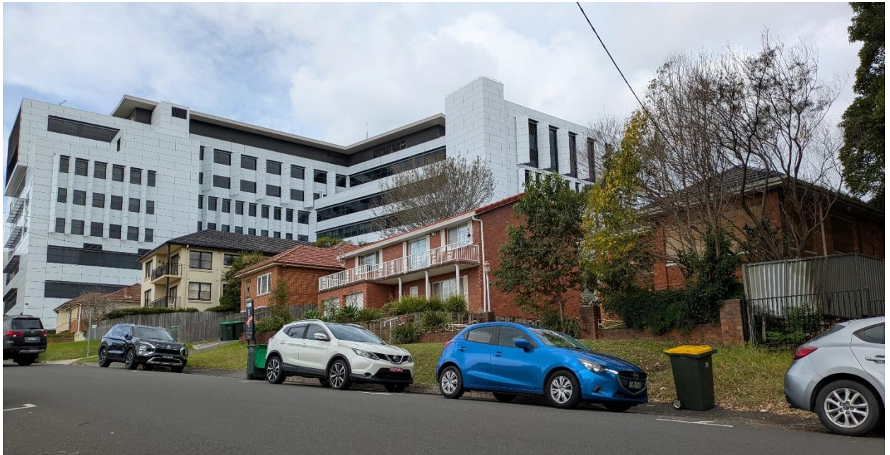
Figure 8 Existing private hospital building (at left) and Nos. 15, 17, 19, 21, and 23 Urunga Parade & 360-364 Crown Street, viewed from Urunga Parade.
