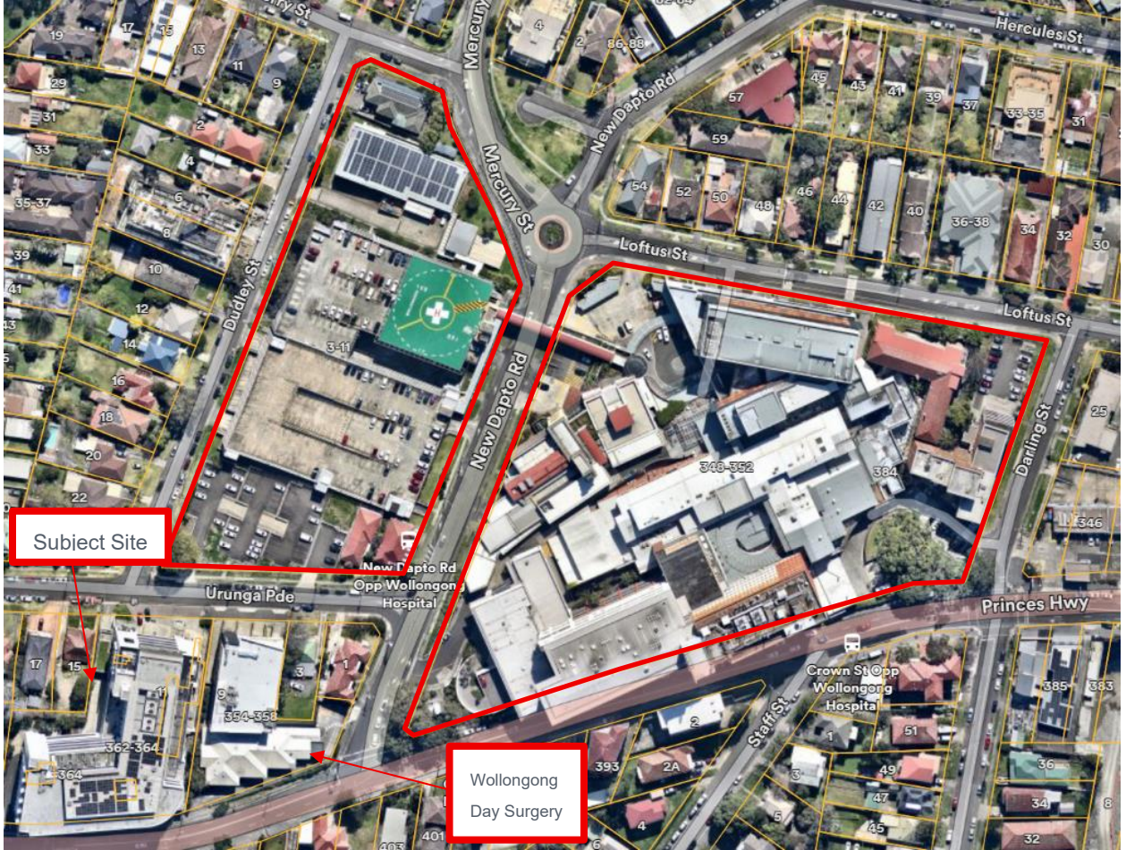
Figure 17 Wollongong Public Hospital (Source: NearMaps 2025).
