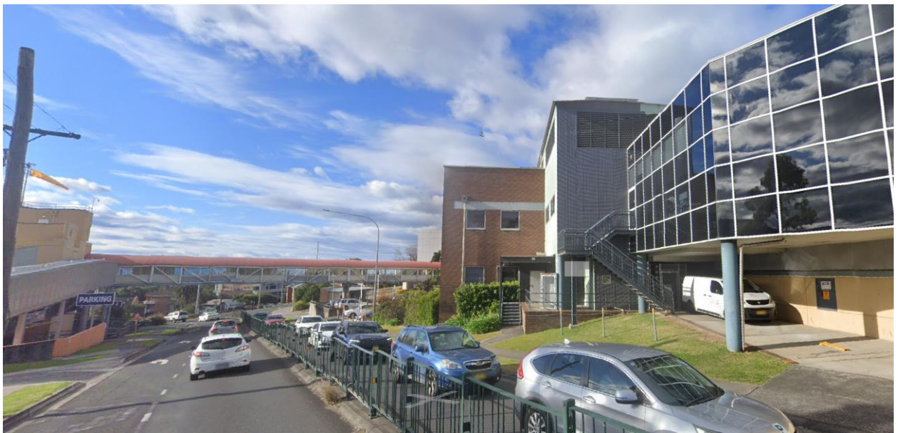
Figure 21 Wollongong Public Hospital, as viewed from New Dapto Road.
