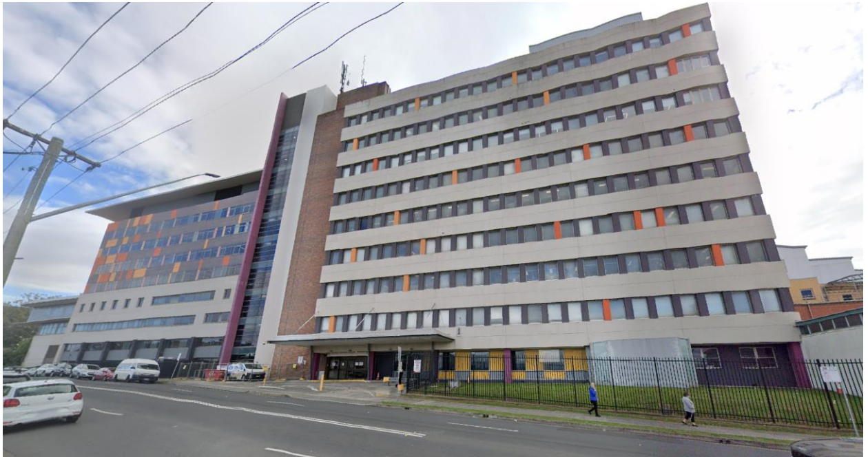
Figure 18 Wollongong Public Hospital, as viewed from Crown Street.
