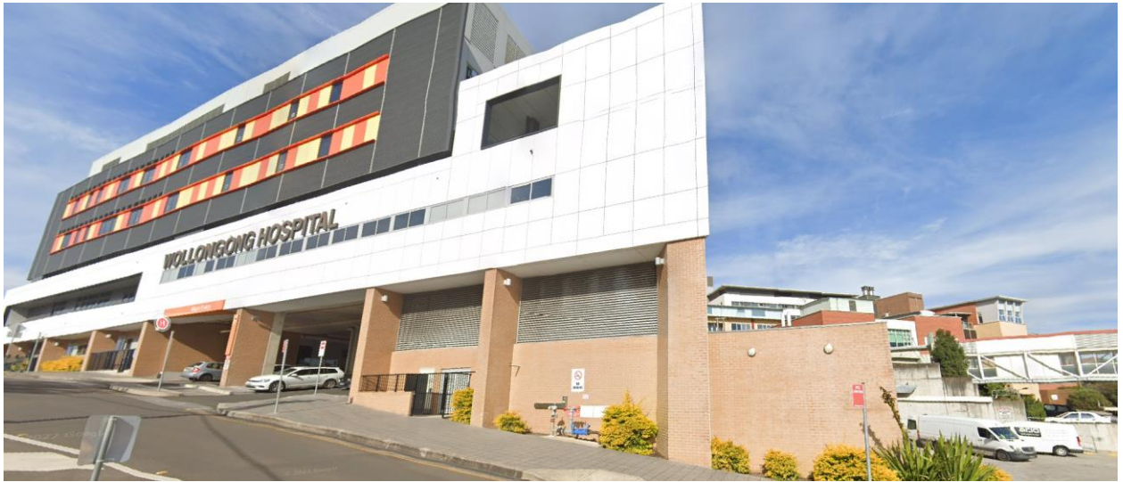
Figure 20 Wollongong Public Hospital, as viewed from Loftus Street.
