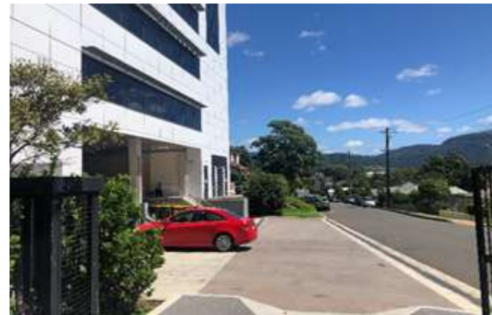
Urunga Parade loading dock view
