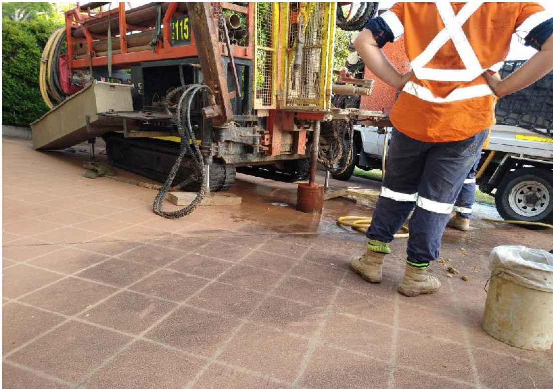
Photo 1: Concrete coring of Bore 301.
