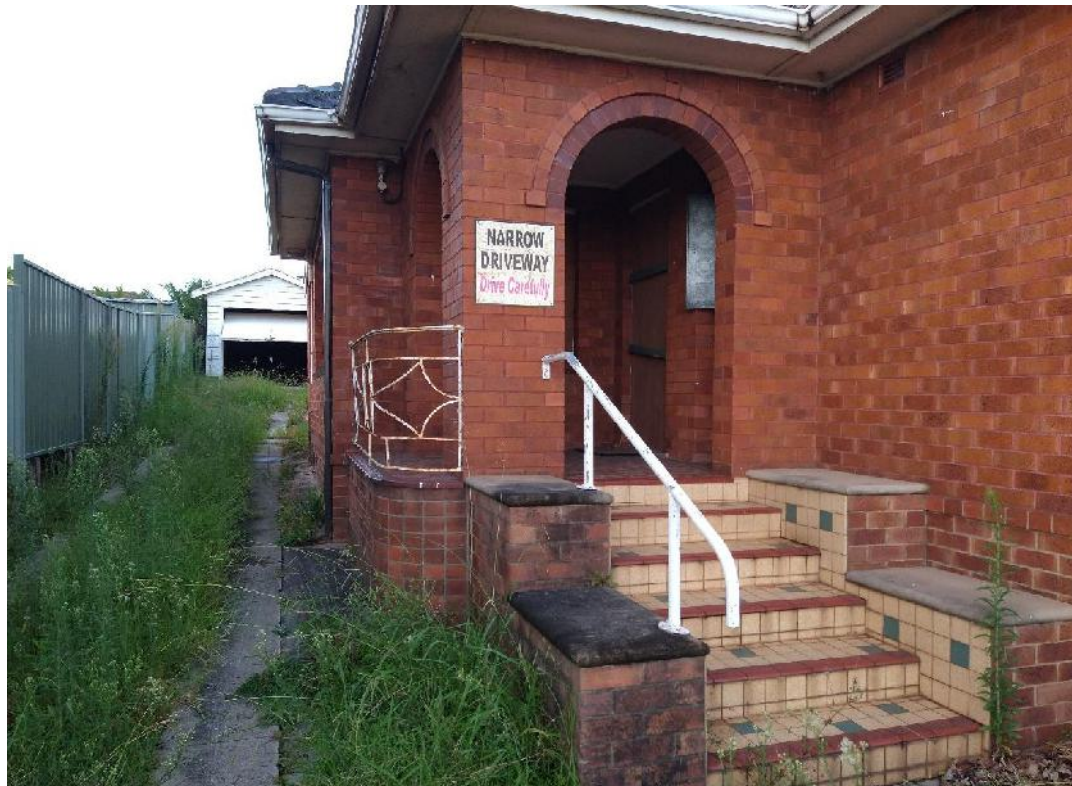
Photo 5: General view of No. 23 Urunga Parade driveway and residential entrance, looking south.
