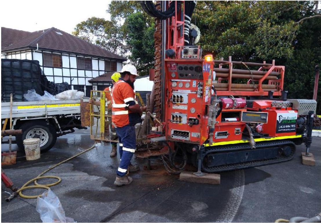
Photo 2: General view of drillers augering through natural material, Bore 303.
