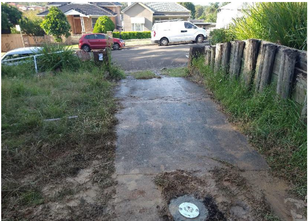
Photo 8: General view of Bore 401 with groundwater monitoring well installed after drilling, looking north.
