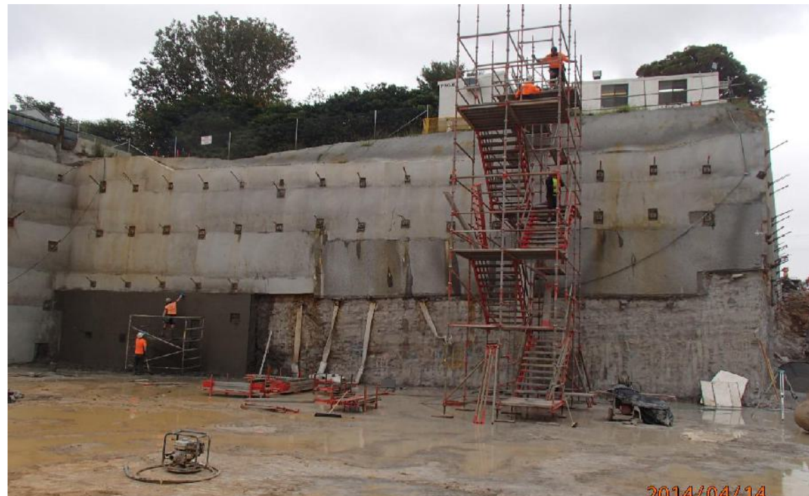
Photo 15: View looking north toward the fifth bench of the Wollongong Private Hospital excavation adjacent to the rear boundary of No. 15 and 17 Urunga Parade. Note: this is the design (ie completed) basement excavation level.
