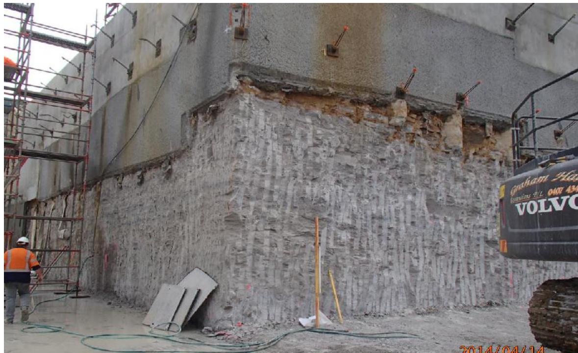
Photo 16: View looking north west toward the fifth bench of the Wollongong Private Hospital excavation adjacent to the south eastern corner of No. 15 Urunga Parade. Note: this is the design (ie completed) basement excavation level.
