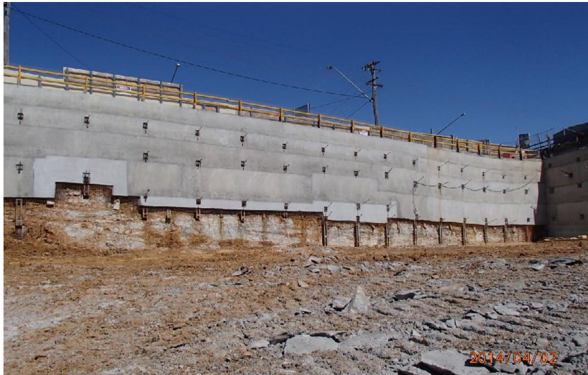
Photo 13: View looking south west toward the fifth bench of the Wollongong Private Hospital excavation adjacent to Crown Street. Note: this is the design (ie completed)
