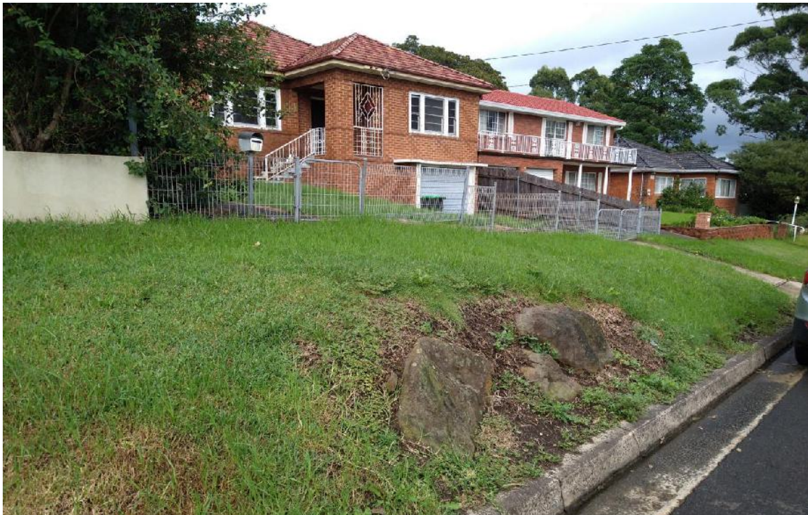
Photo 5: View looking at medium strength sandstone blocks exposed in the nature strip at the front of No. 17 Urunga Parade.
