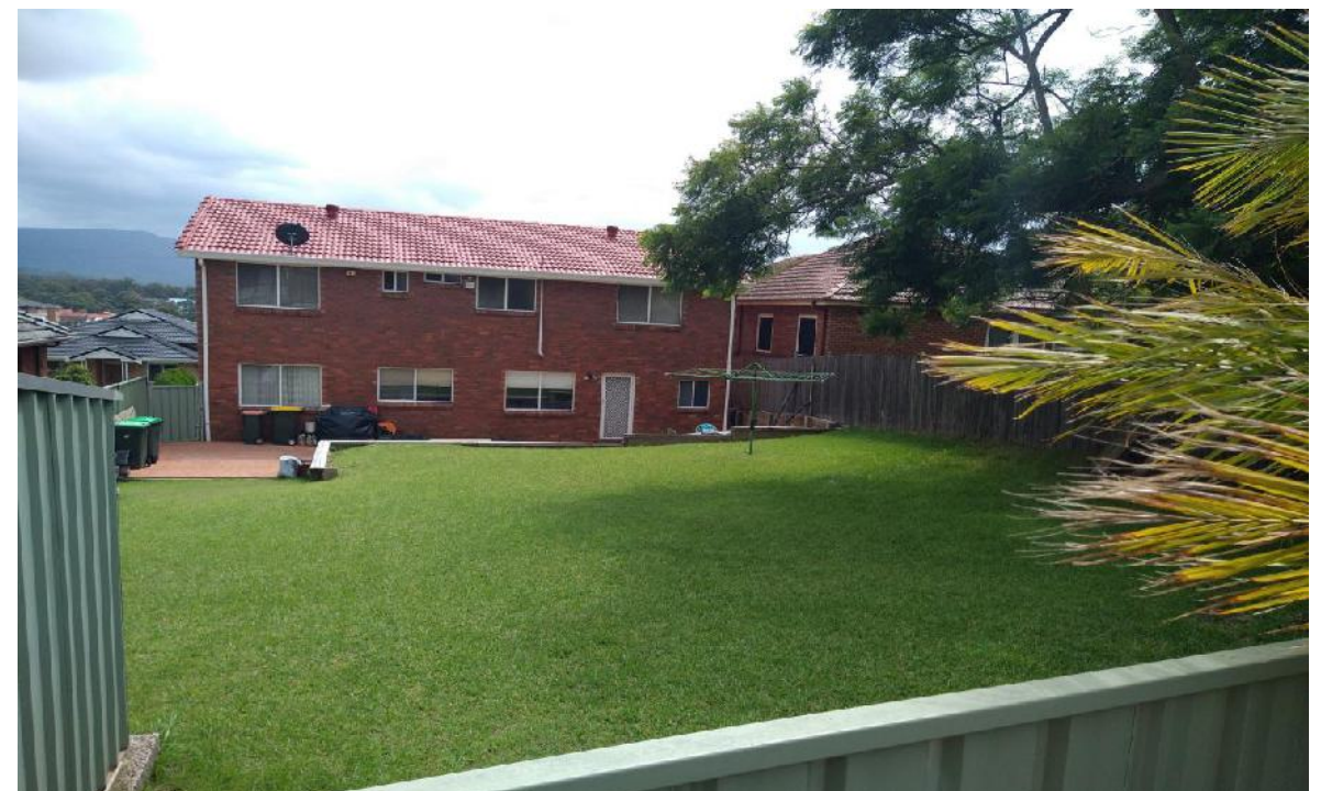
Photo 8: View looking north at the backyard of No. 21 Urunga Parade.
