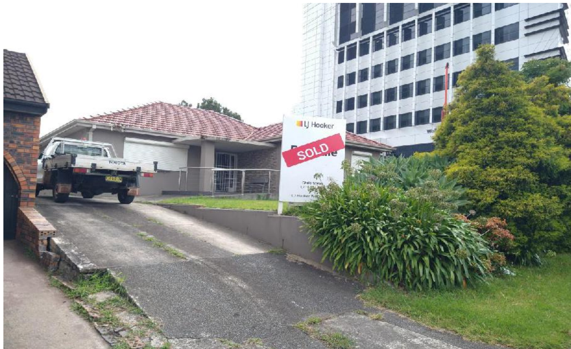
Photo 7: View looking north east towards No. 368 Crown Street.
