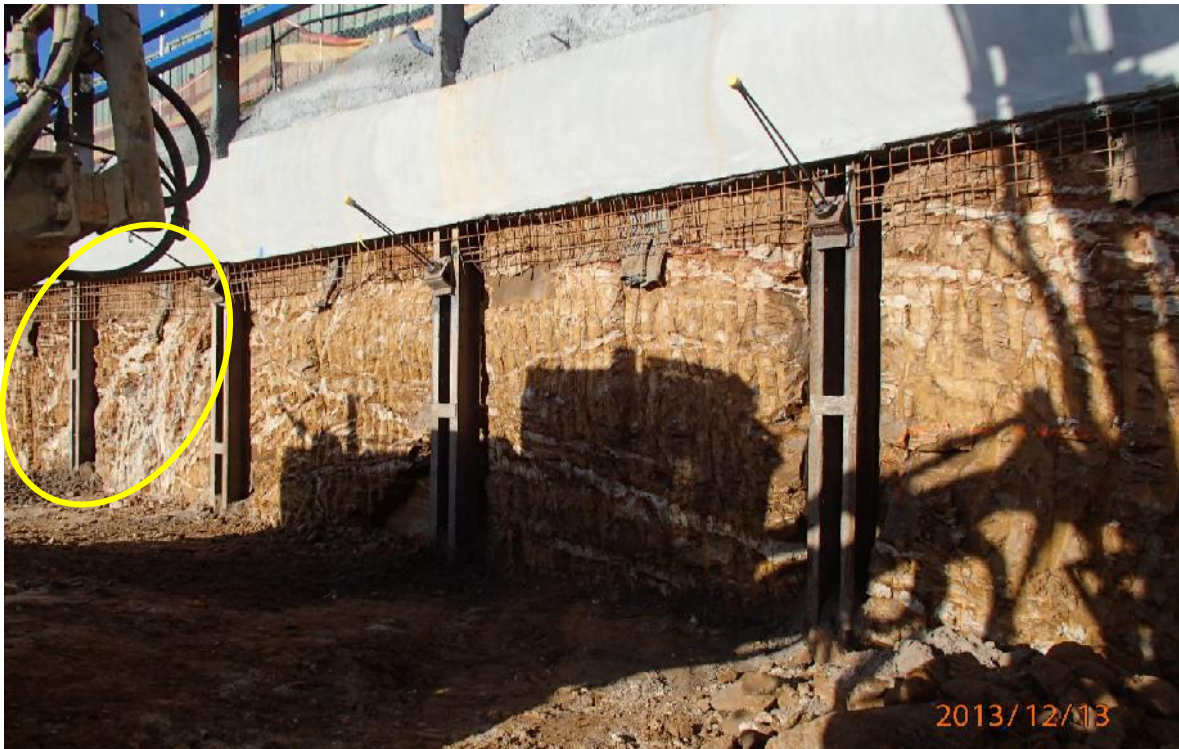
Photo 10: View looking south east at the weathered sandstone profile exposed in the second bench of the Wollongong Private Hospital excavation, adjacent to Crown Street.
