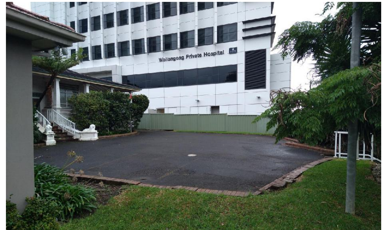
Photo 4: View looking east across the front of No. 366 Crown Street. Note: Bore 304 in the centre of the photo.
