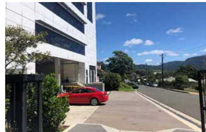
Urunga Parade loading dock view
