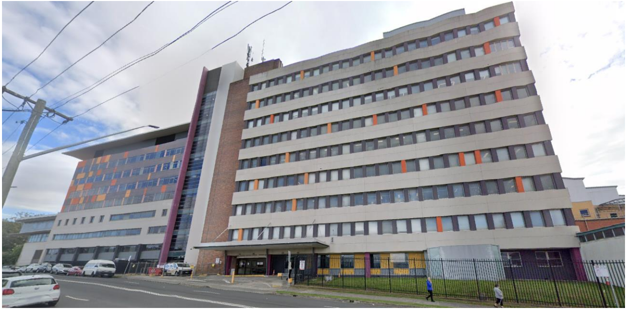
Figure 4 Wollongong Public Hospital, as viewed from Crown Street.
