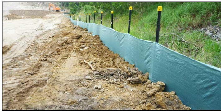
Figure 3: Sediment Fence (example)
