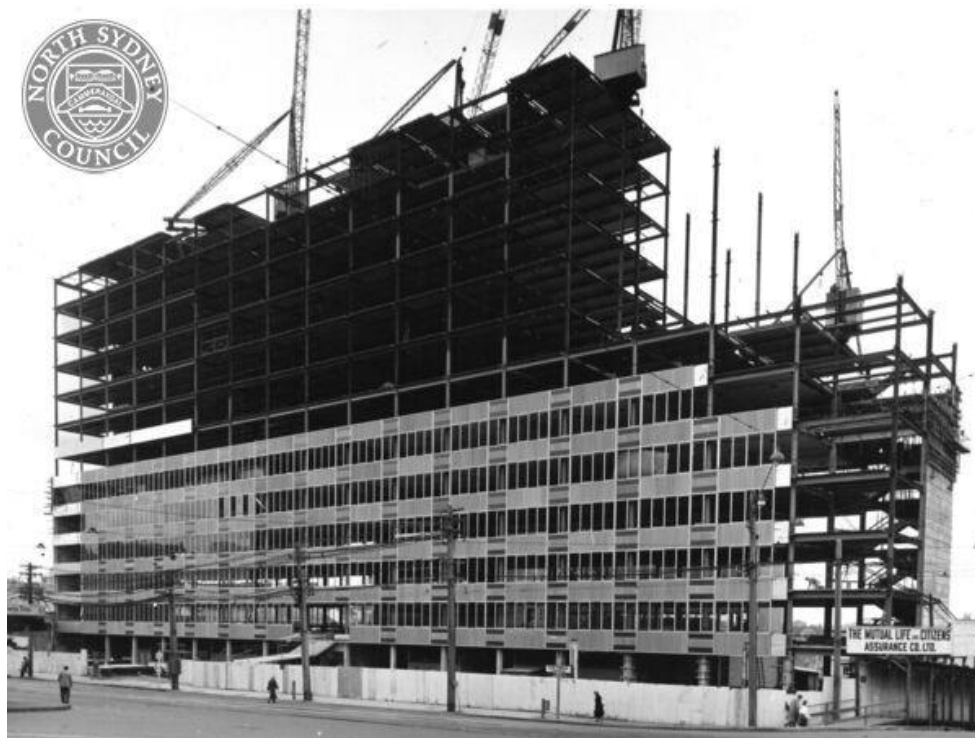
Figure 4-9: MLC Building under construction in 1956.
