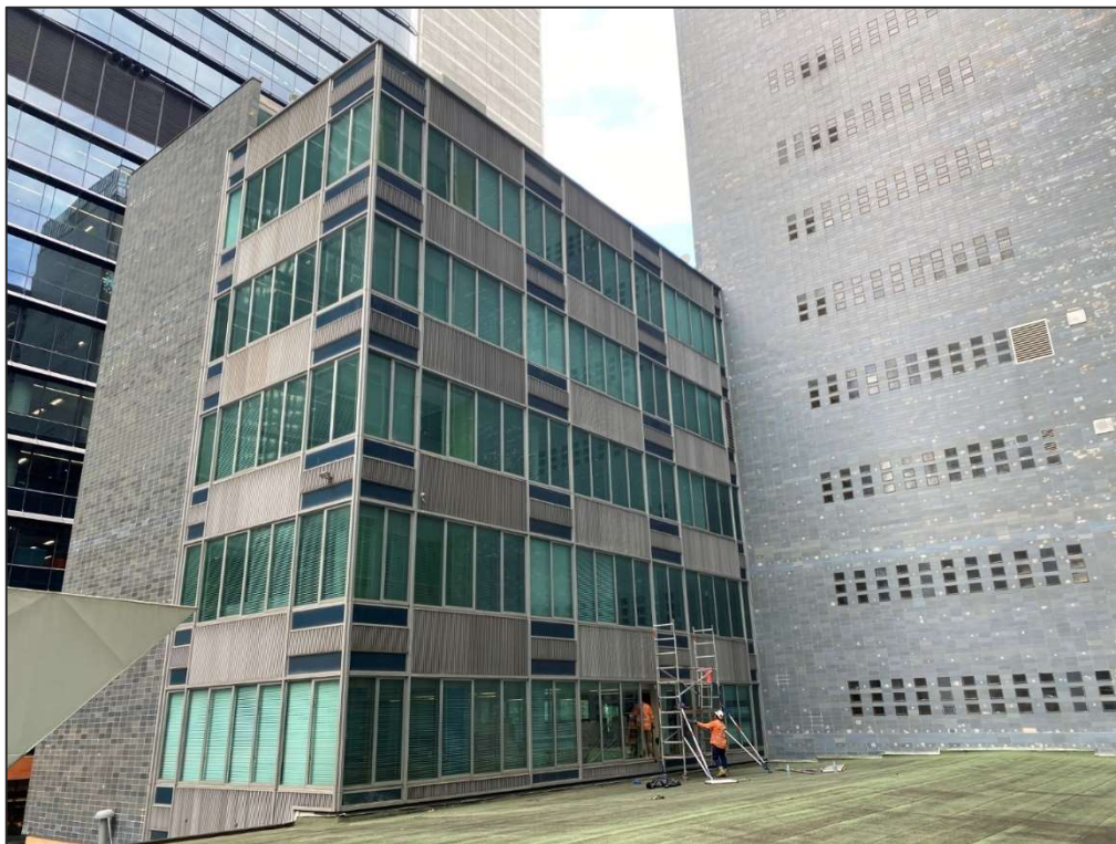
Photograph 4: Scaffolding was erected on the northern ground level rooftop to access the external façade.
