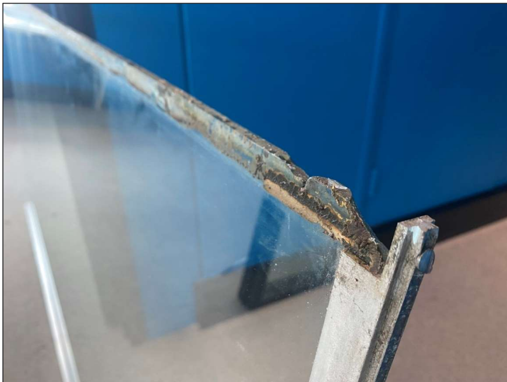
Photograph 2: Inner vision windows were removed, and sealant materials around glazing sampled. All collected samples were analysed for asbestos analysis by a NATA accredited laboratory.
