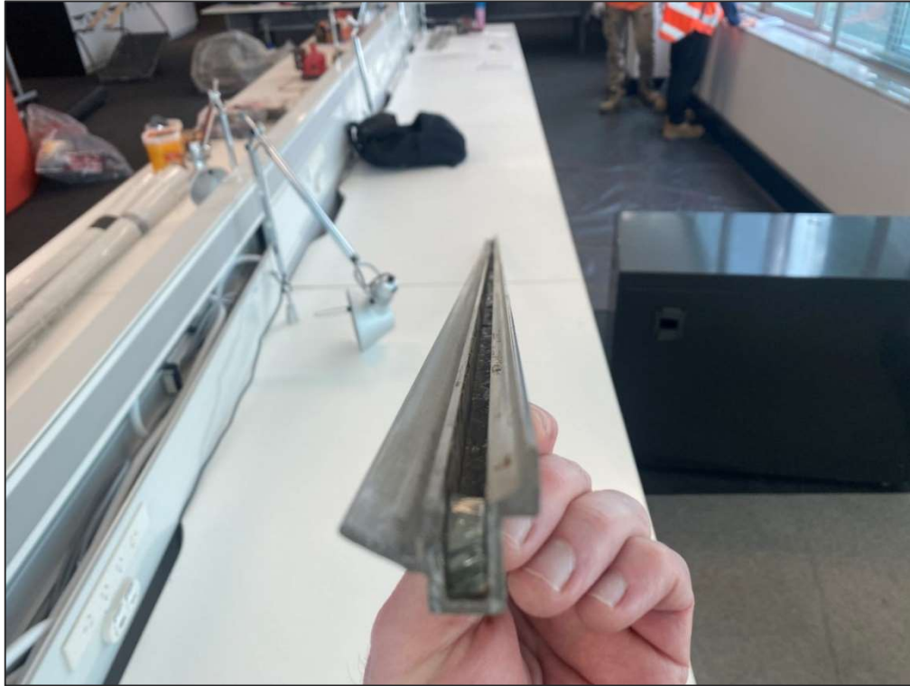
Photograph 3: Glazing channel of inner vision windows.
