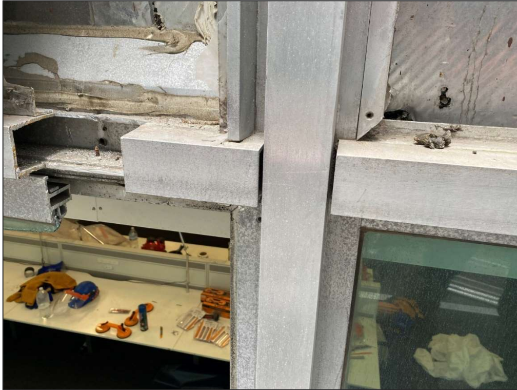
Photograph 11: Front view of mullion / head transom connection to the curtain wall.
