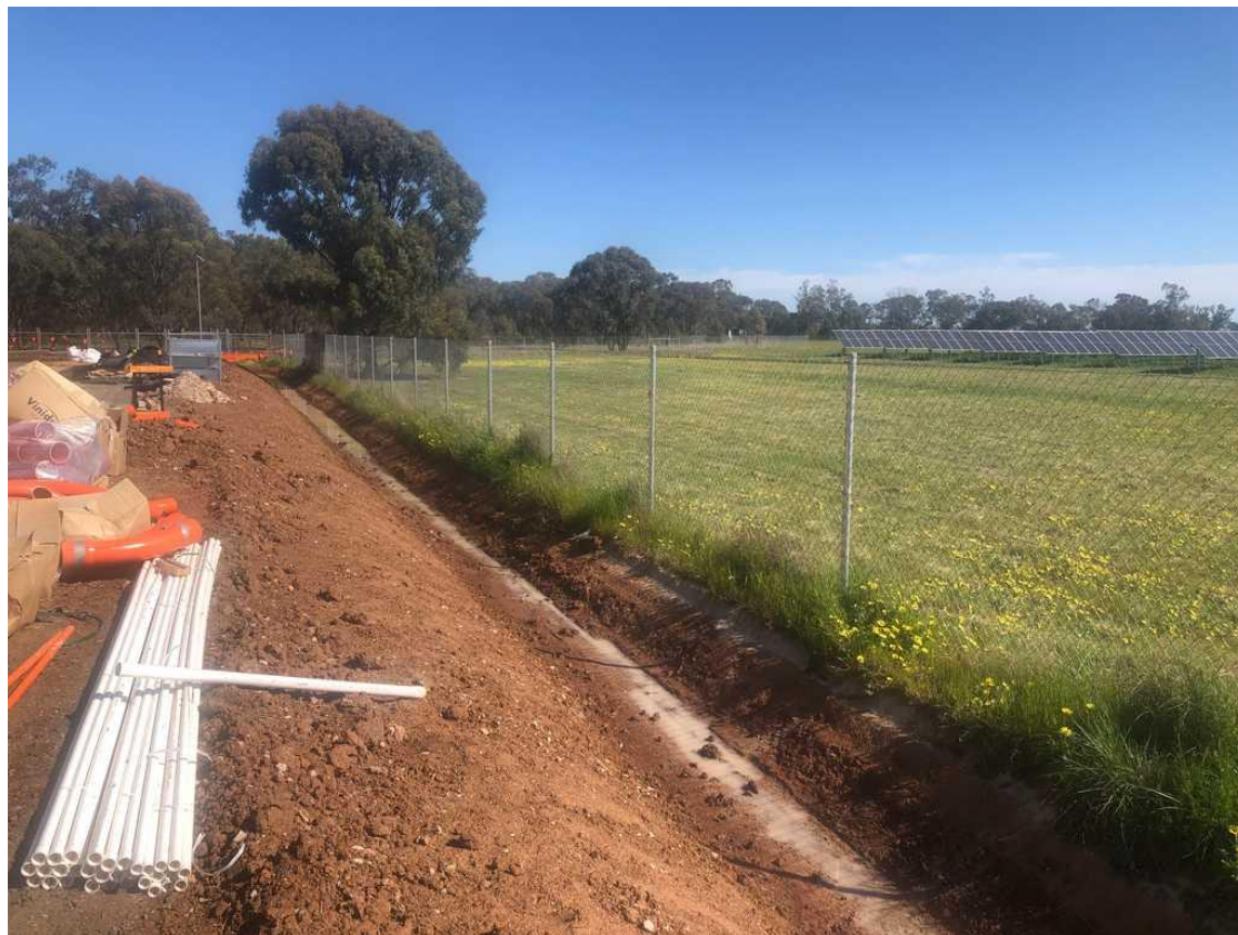
Photos 4 – Utilisation of Catch Drains to Capture Runoff From Disturbed Areas and Direct Runoff into Evaporation Pond. Batter treatment Recommended Along Diversion Drain
