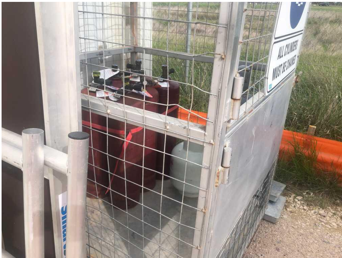
Photo 14 – Oxyacetylene Cylinder in caged compartment
