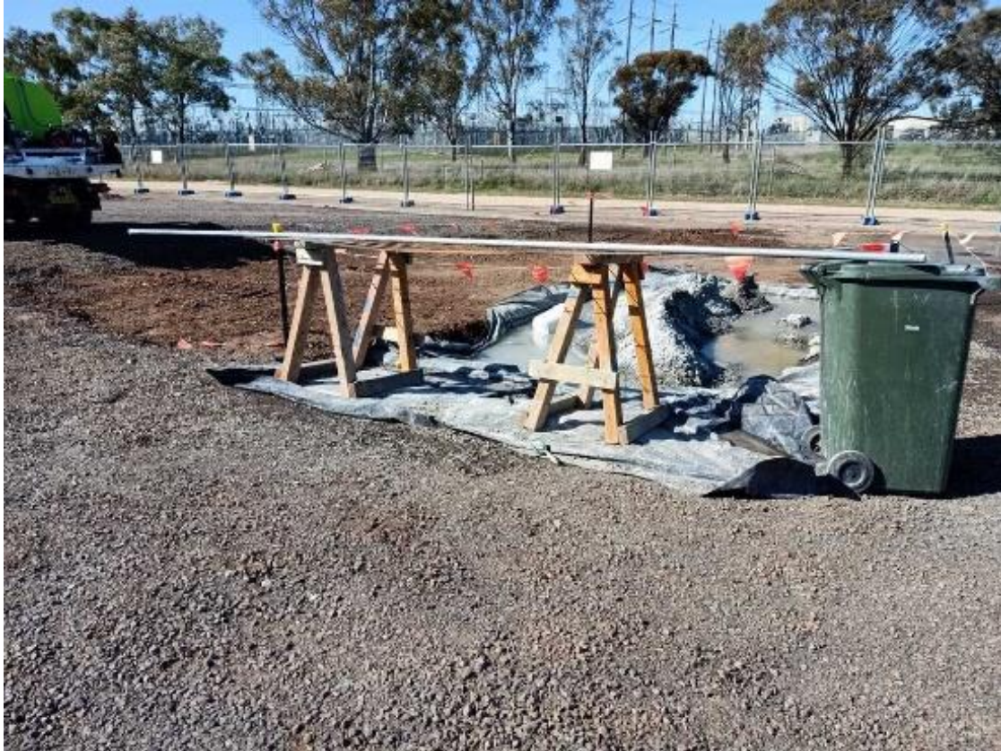
Photo 9(a) – Concrete washout pit with lining material – requires maintenance
