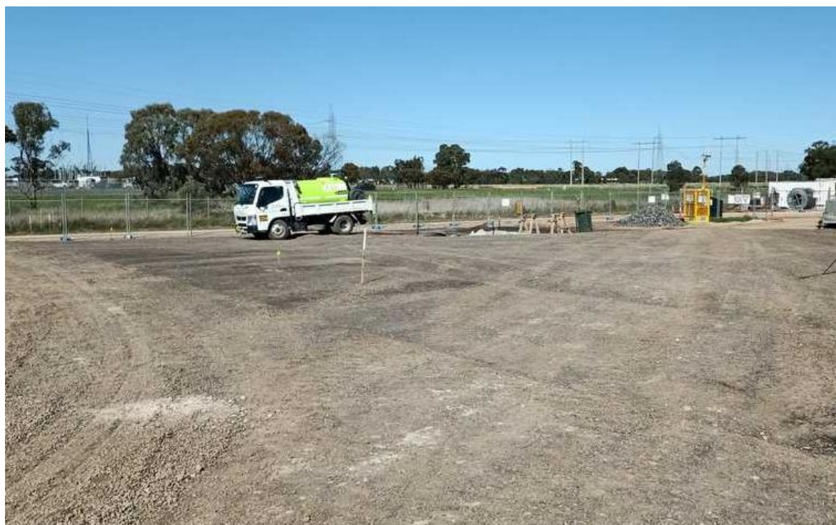
Photo 6(f) – Water cart in operation for dust suppression
