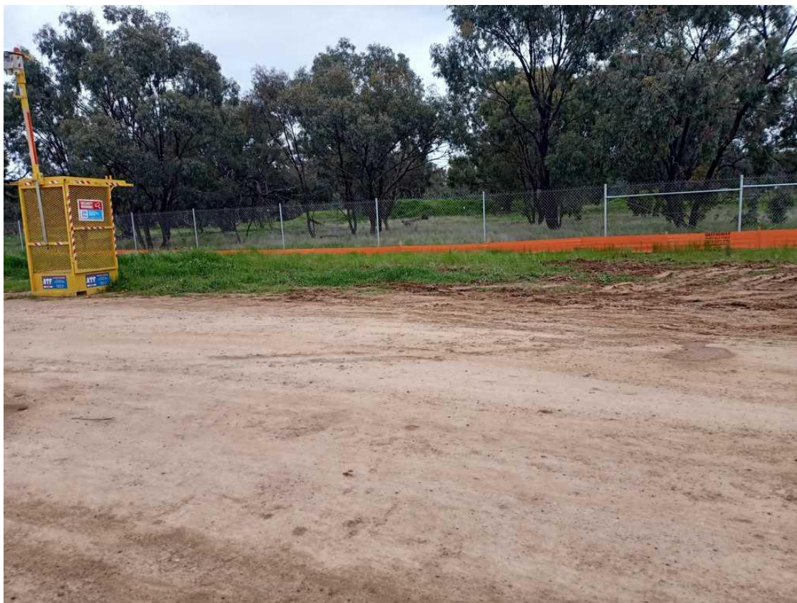
Photo 8(b) – Sediment fence installed along site boundary
