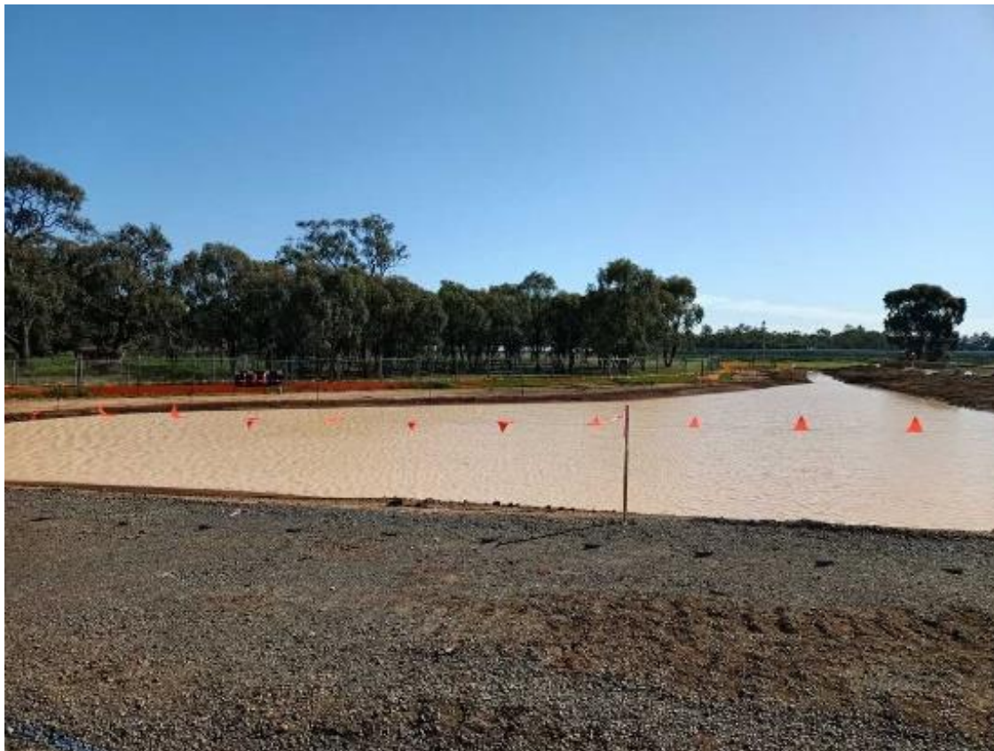
Photo 8(c) – Utilisation of Evaporation Pond to Capture Runoff from Disturbed Areas
