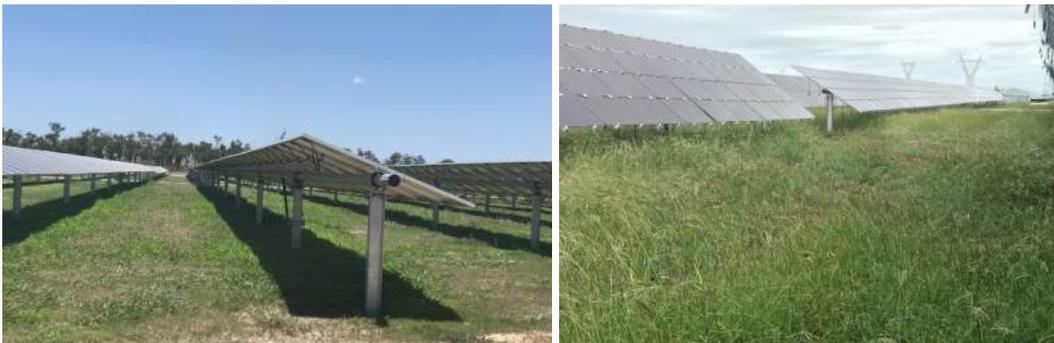
Photograph 6 Example of grassland rehabilitation between and under panels within 2 to 4 weeks after completion of construction of solar arrays
