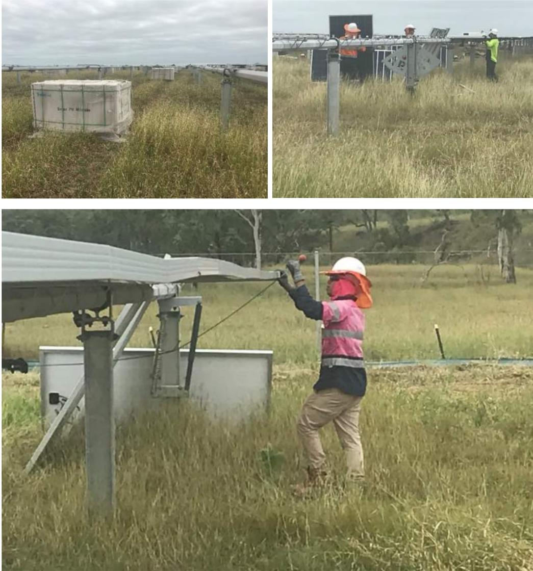
Photograph 4 Module installation
