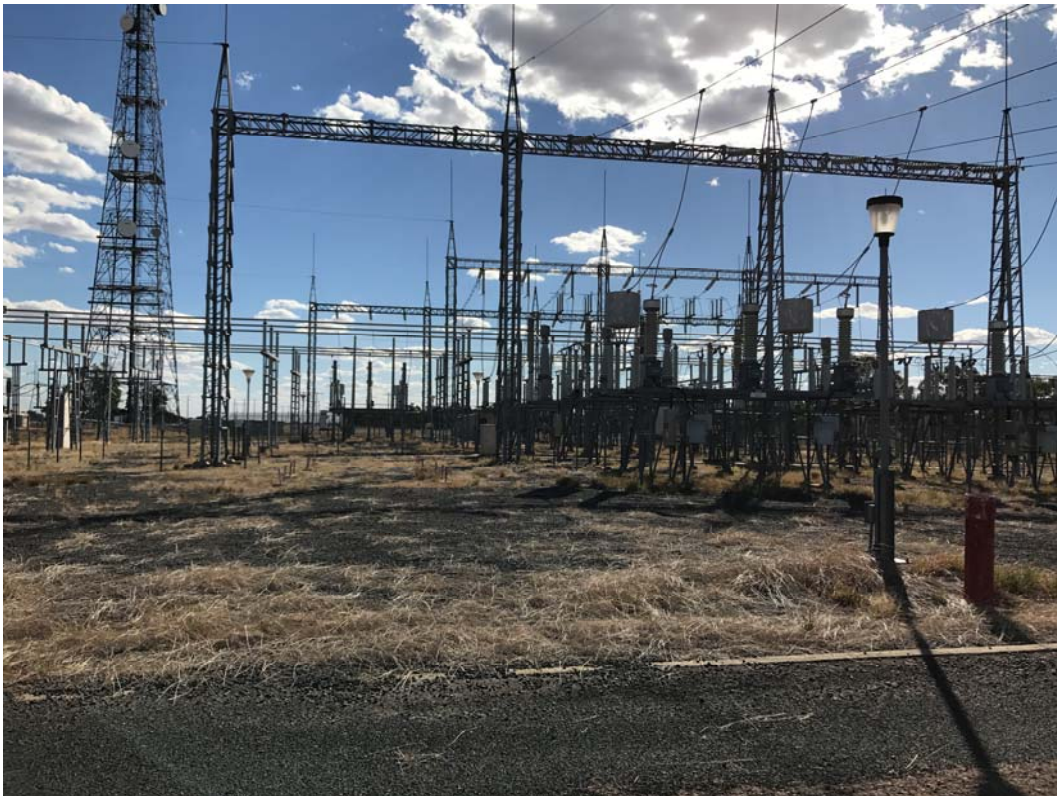
Photograph 4 At the TransGrid substation showing the spare 132 kV bay and gantry
