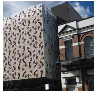
Koori radio station building, TZG
