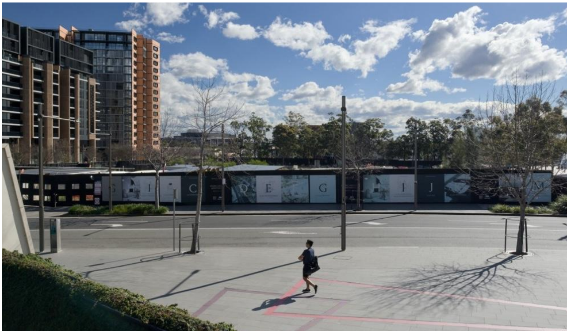
Green Square site
