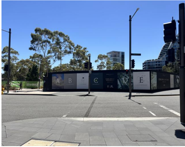
Figure 2 The site viewed from Paul St and Zetland Ave
