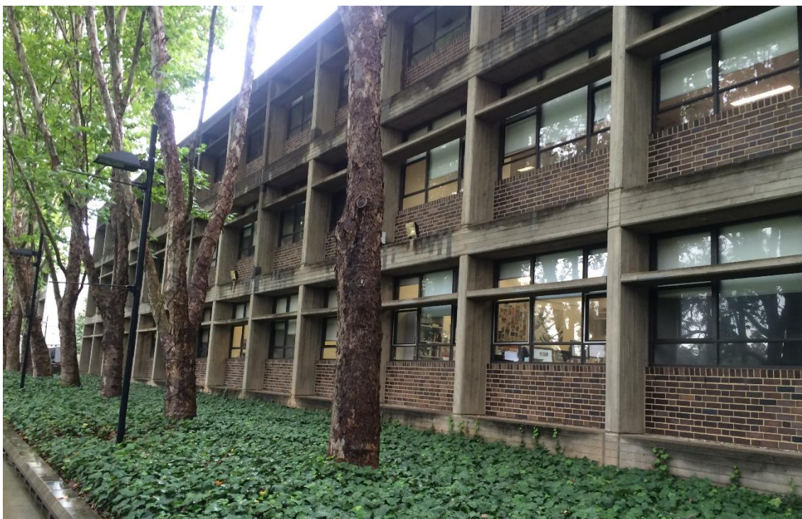
Figure 4 – Building known as W6B, northern elevation
