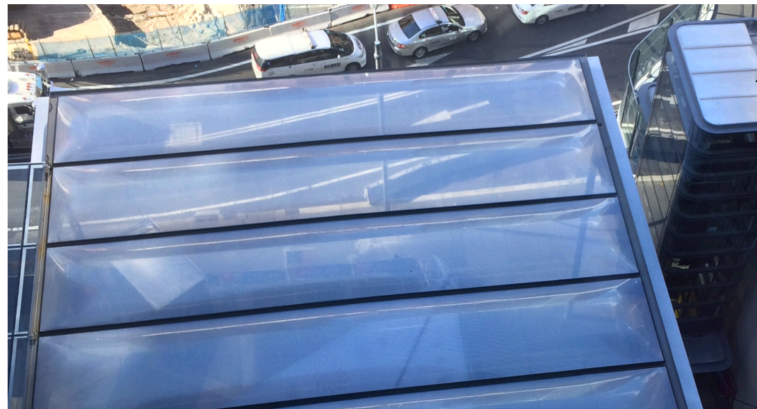
ETFE roof - view from above
