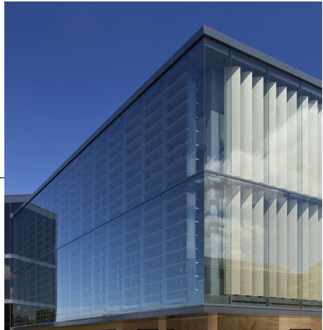
Glazed twin wall facade with integral aluminium sun shade louvers
