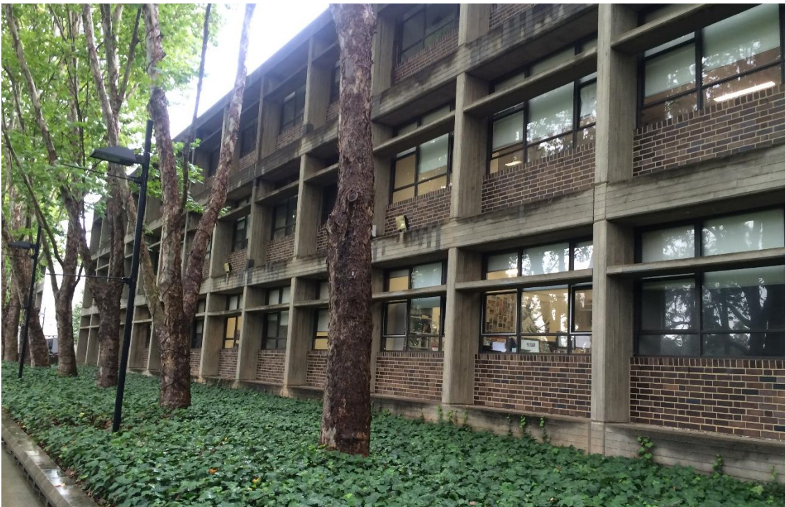
Figure 4 - Building known as W6B, northern elevation
