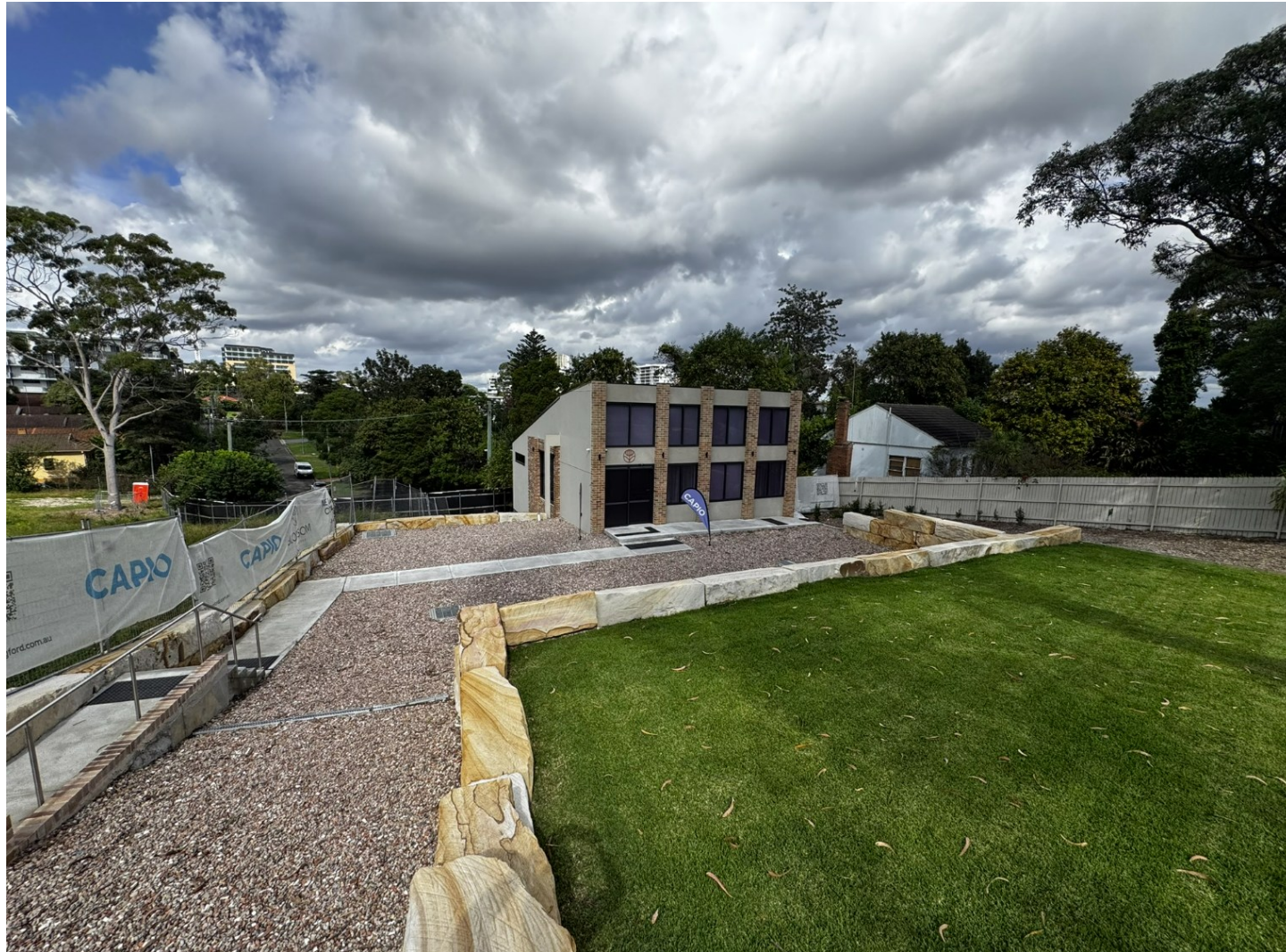
Photograph 11: View South from Moseley Street towards existing built surfaces and planted native trees within north-western portion of the Subject Site
