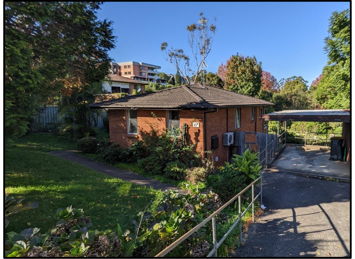
Figure 17. Overall view of the property at No. 15B Moseley Street.
