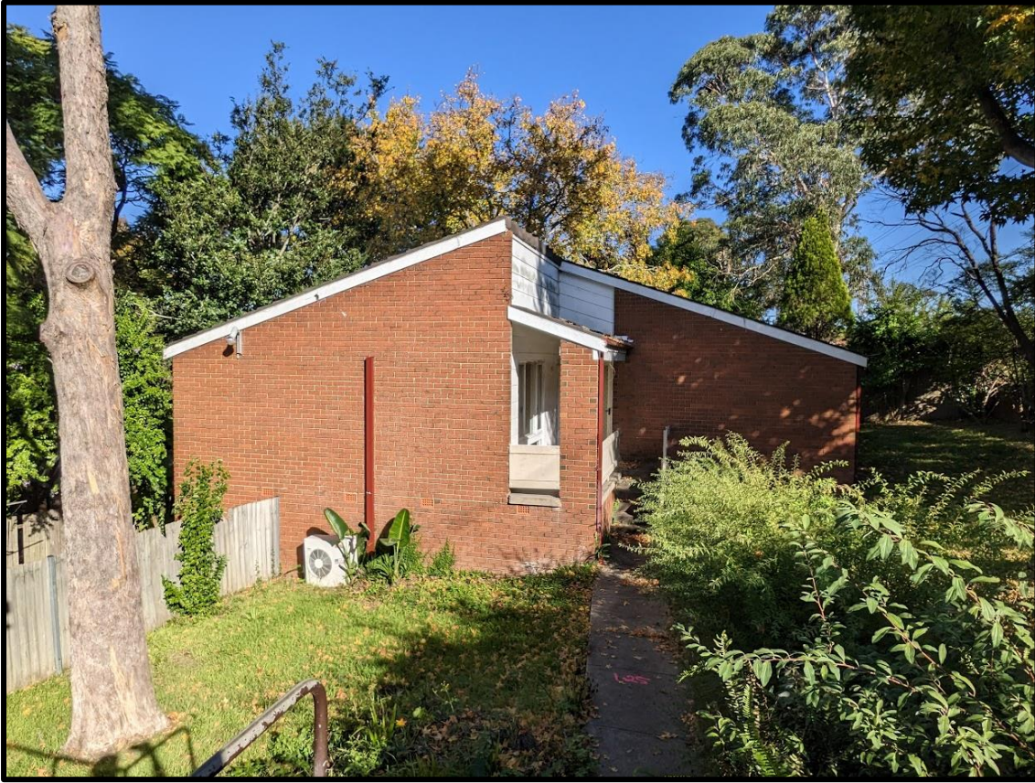
Figure 16. Brick dwelling within the property at No. 15A Moseley Street.
