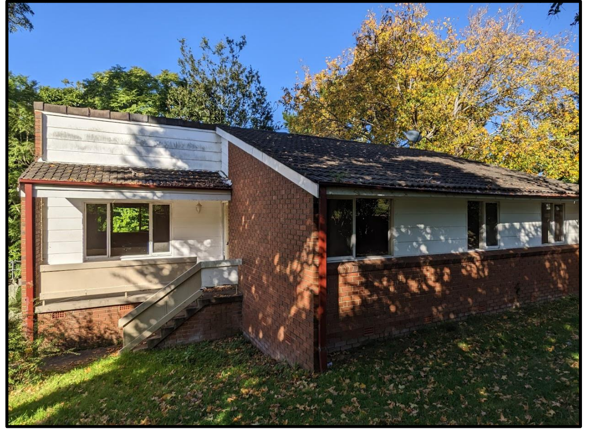
Figure 21. Mixed brick and weatherboard dwelling within the property at No. 15A Moseley Street.
