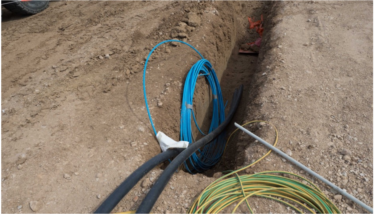
Figure 22: Trenches and for underground cabling
