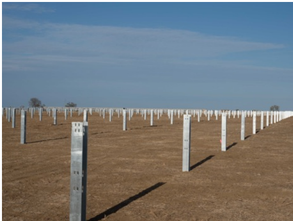
Installed "H" beam piles
