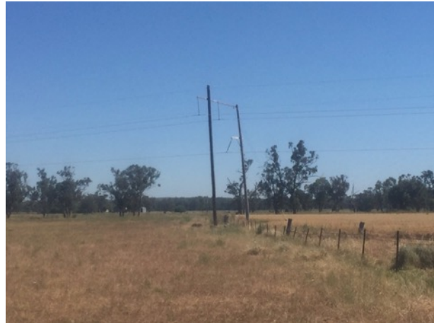
Photo 2: 132kV Powerline crossing site corner
