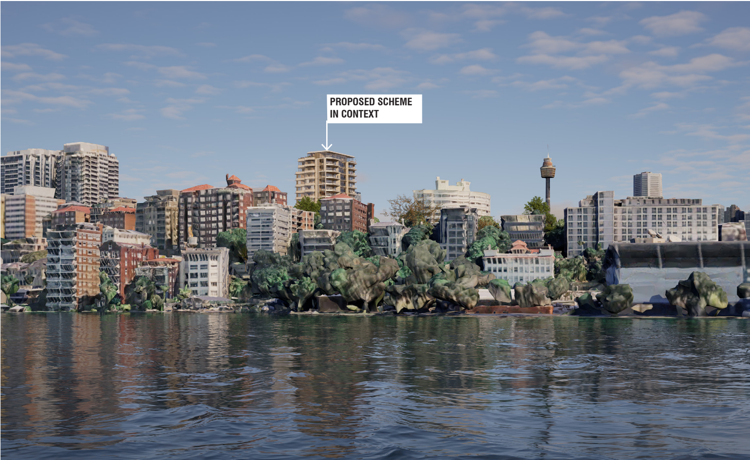
Building in context from Elizabeth Bay
