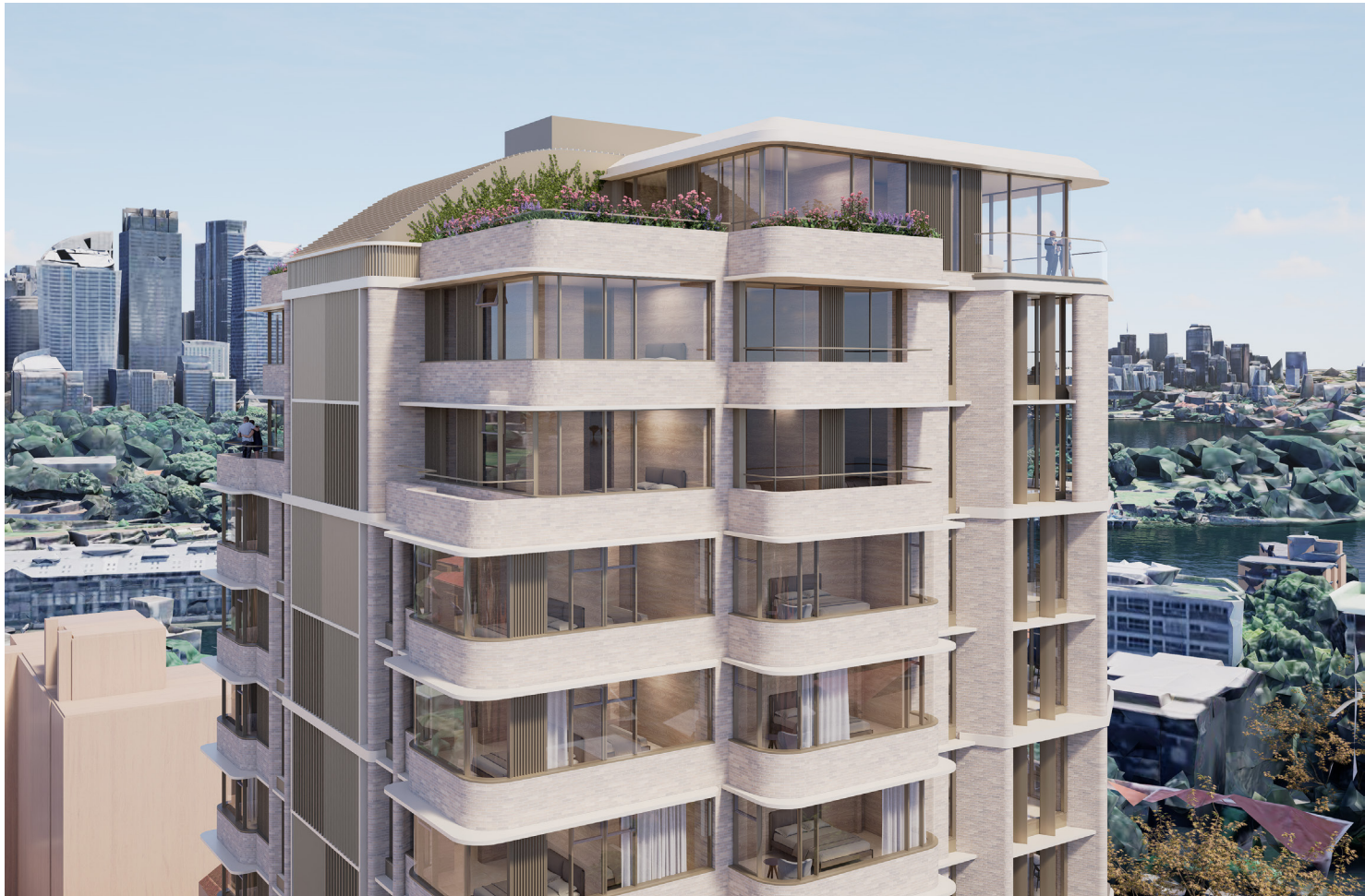
Sub-penthouse set in on southern side
