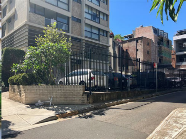
Figure 13 – View from McDonald Street to north-western side of property
