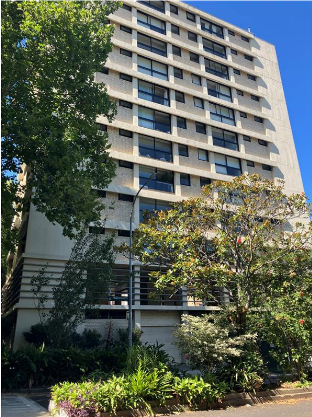
Figure 16 – View south from corner of Macleay and McDonald Streets
