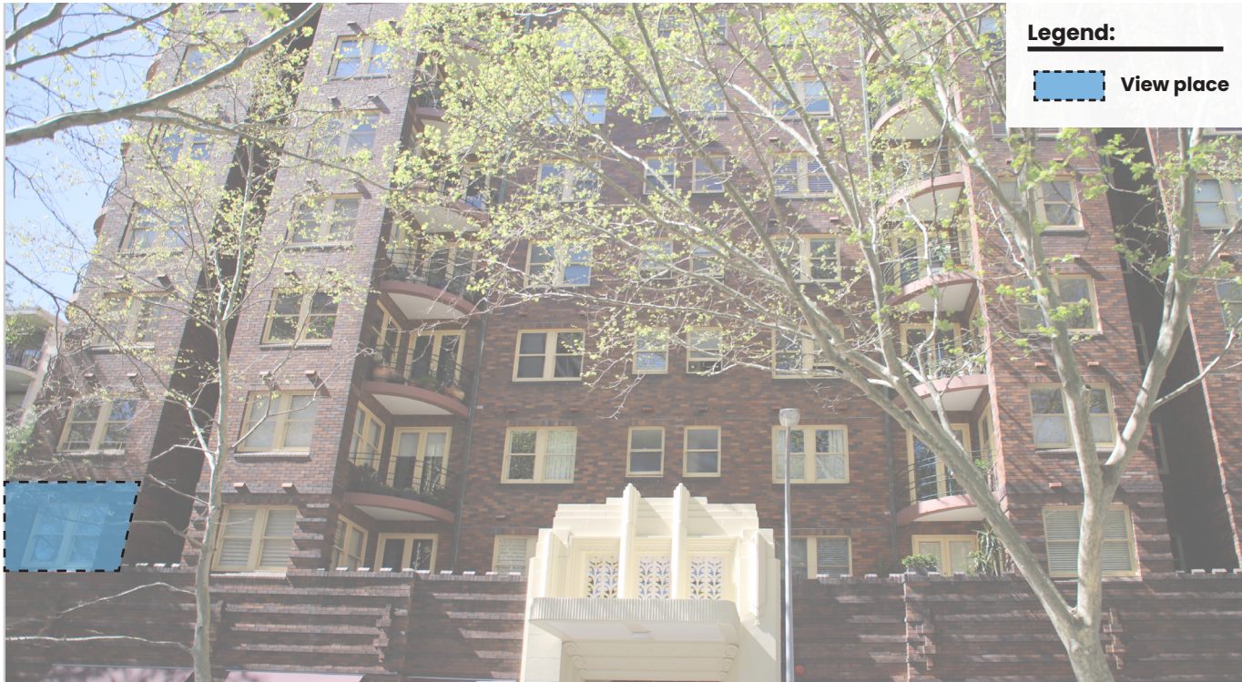
Figure 38 Macleay Regis western elevation, location of Unit 203 indicated in blue.
