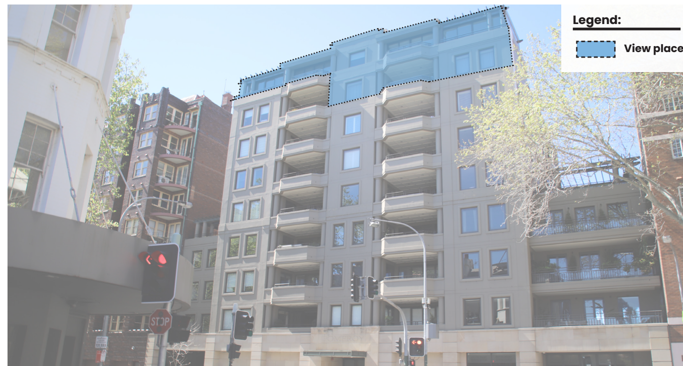
Figure 74 Macleay Regis western elevation, location of Unit 801 indicated in blue.
