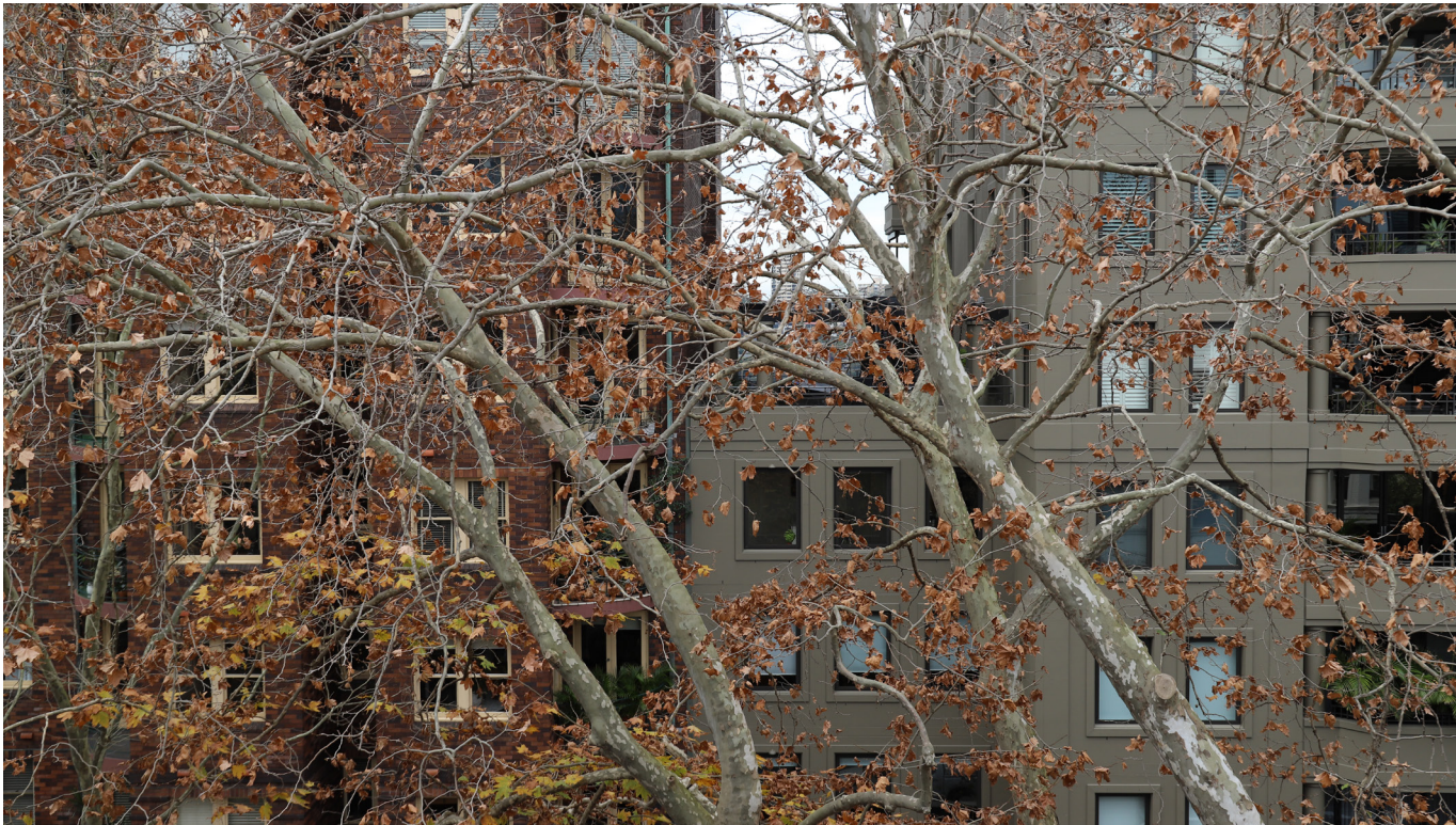
Figure 89 View east (standing) from upper level balcony.
