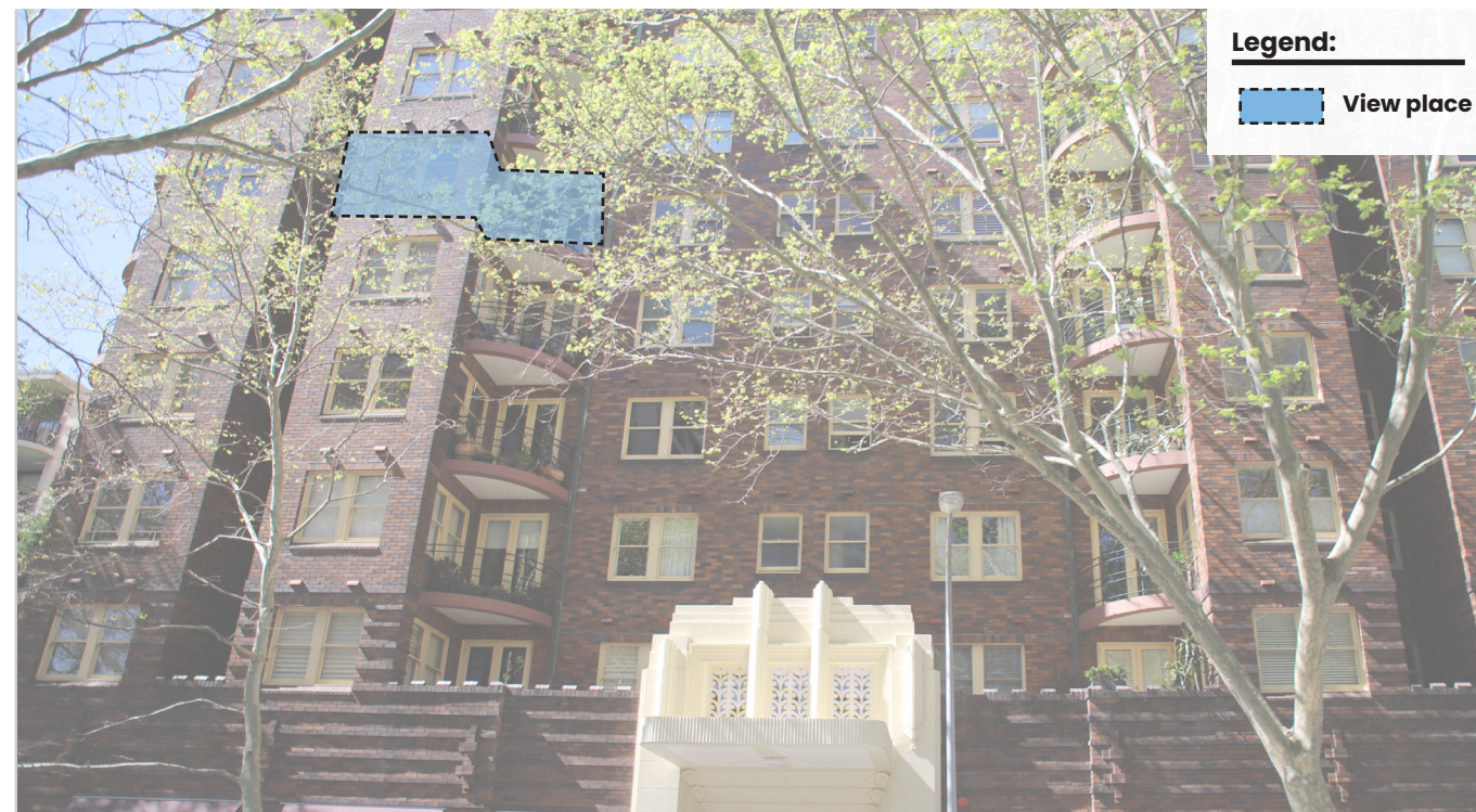
Figure 41 Macleay Regis western elevation, location of unit 602 indicated in blue.
