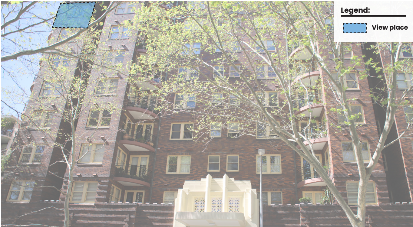
Figure 29 Macleay Regis western elevation, location of Unit 703 indicated in blue.
