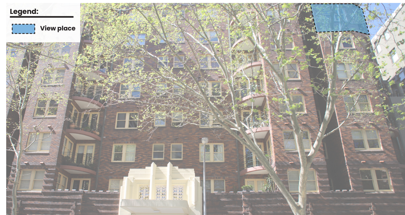
Figure 58 Macleay Regis western elevation, location of Unit 700 indicated in blue.
