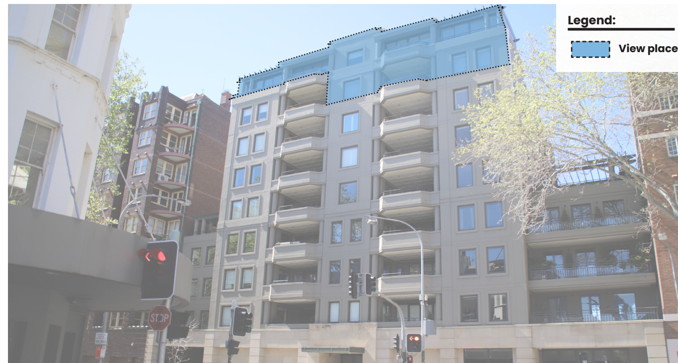
Figure 68 Western elevation of the Pomeroy, location of Unit 801 indicated in blue.
