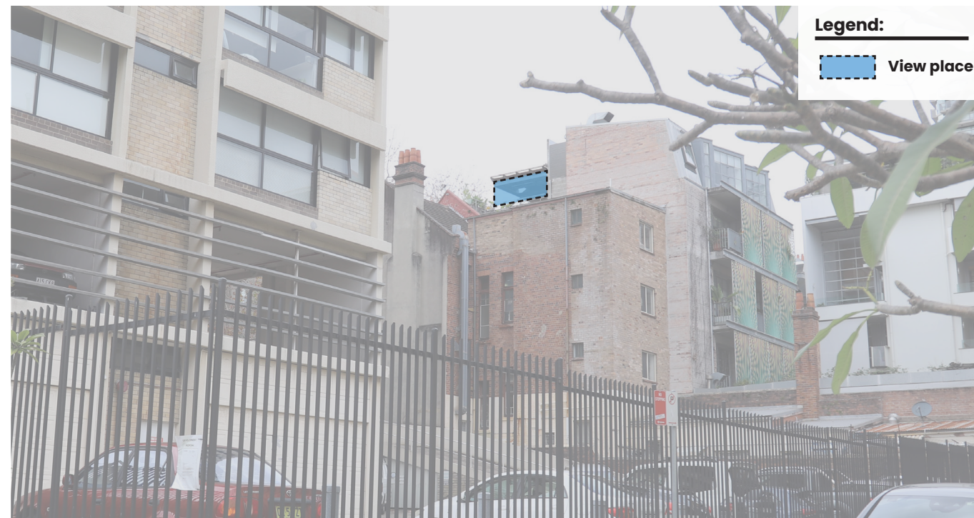
Figure 85 Rear view of Yellow House from McDonald Street towards northern elevation of building, location of Unit 7 balcony indicated in blue.
