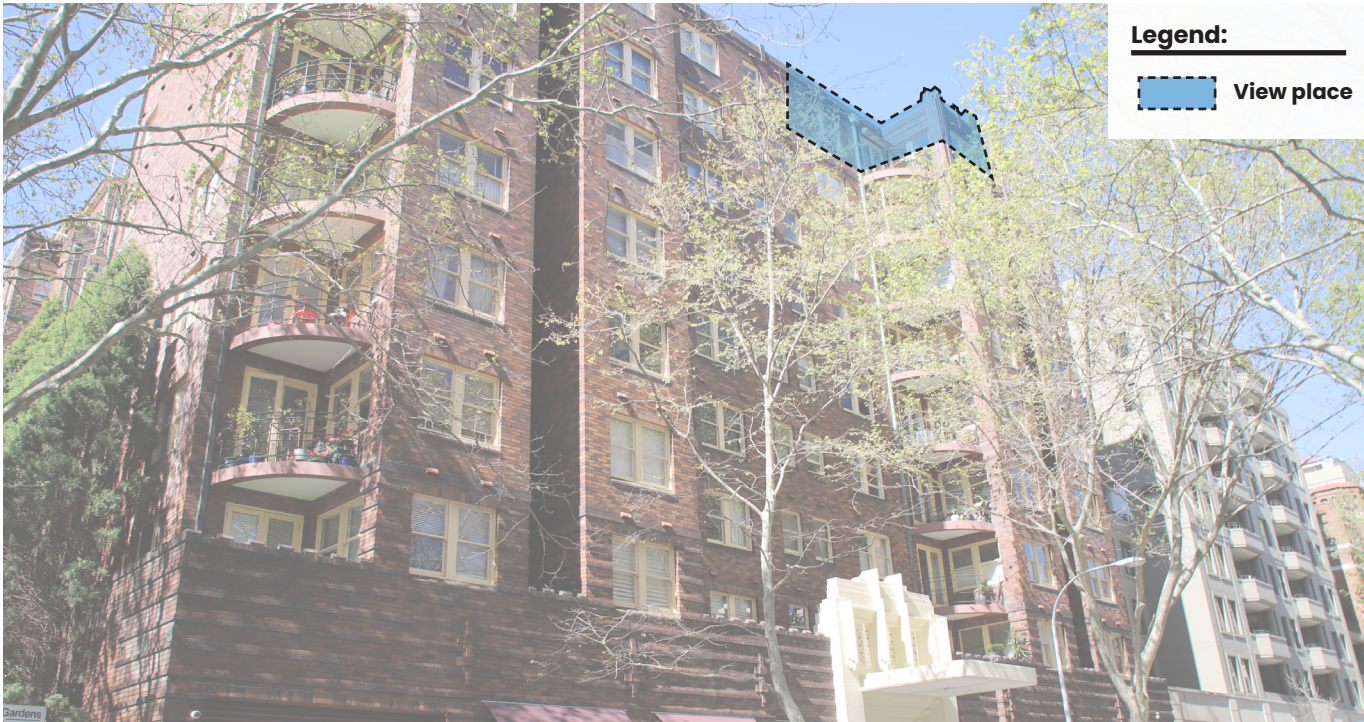
Figure 47 Macleay Regis western elevation, location of Unit 901 indicated in blue.
