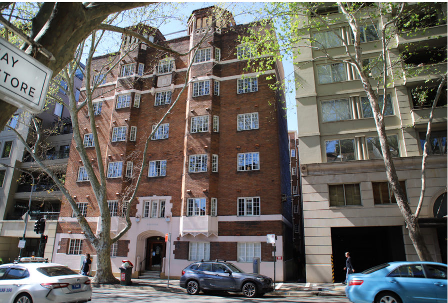
Figure 24 16 Macleay Street (Selsdon).
