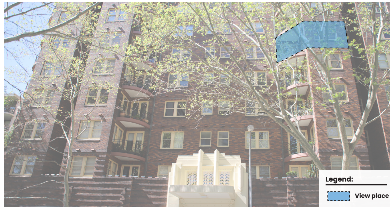
Figure 53 Macleay Regis western elevation, location of Unit 701 indicated in blue.
