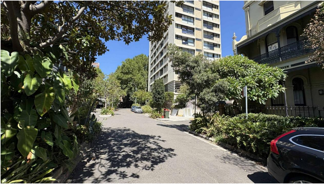
Figure 47 Subject site from McDonald St (subject site on right) (Photo taken: 24/01/2026)
