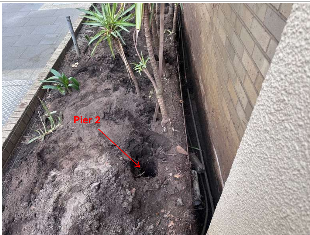
Image 9: The North end of trench 2 and pier 2.
