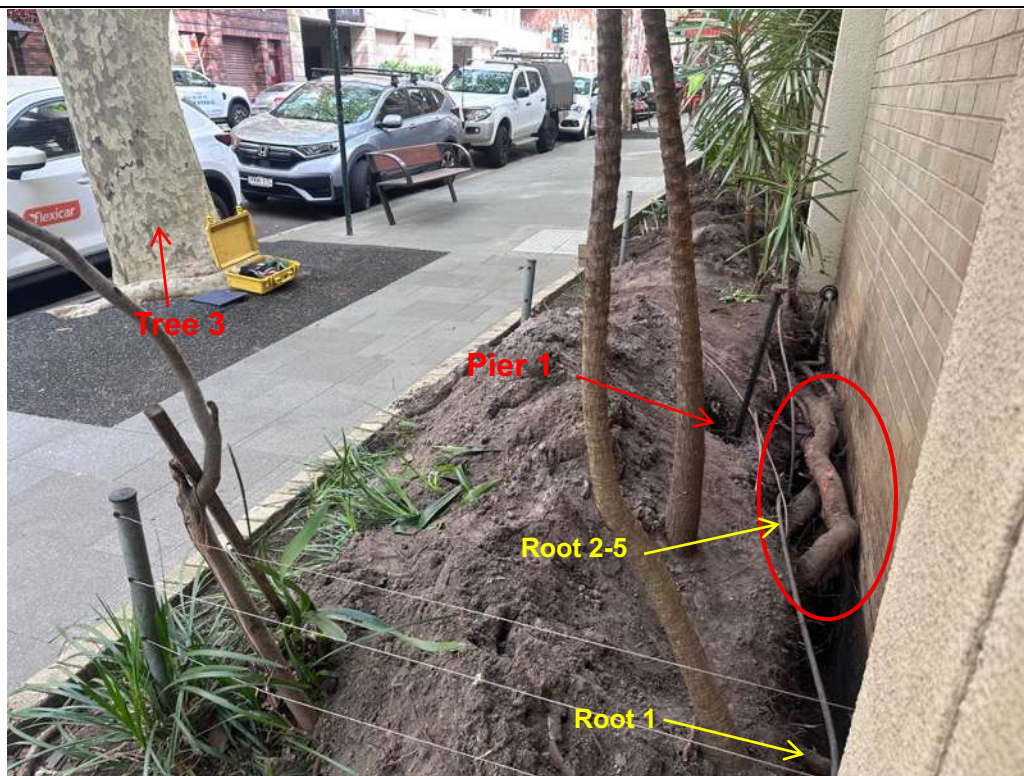
Image 3: Showing the whole of trench 1, the location of pier 1 and the exposed roots in relation to the trunk of tree 3.
