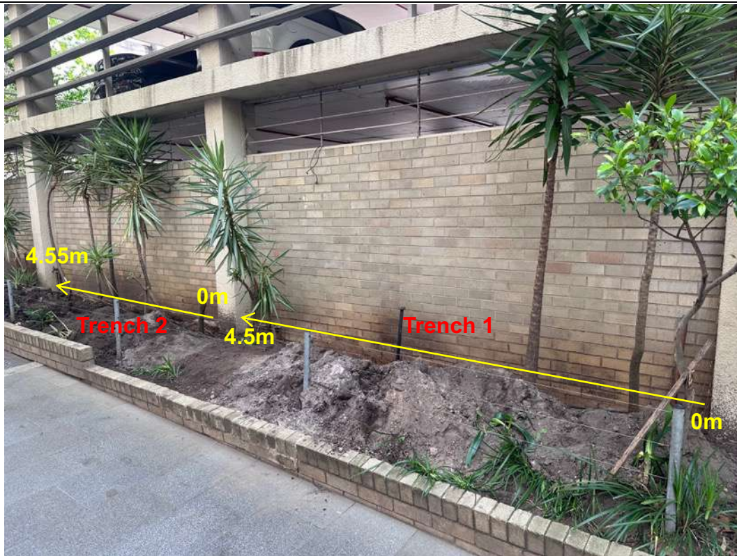
Image 1: Showing the location of trench 1 and 2 either side of the existing columns.
