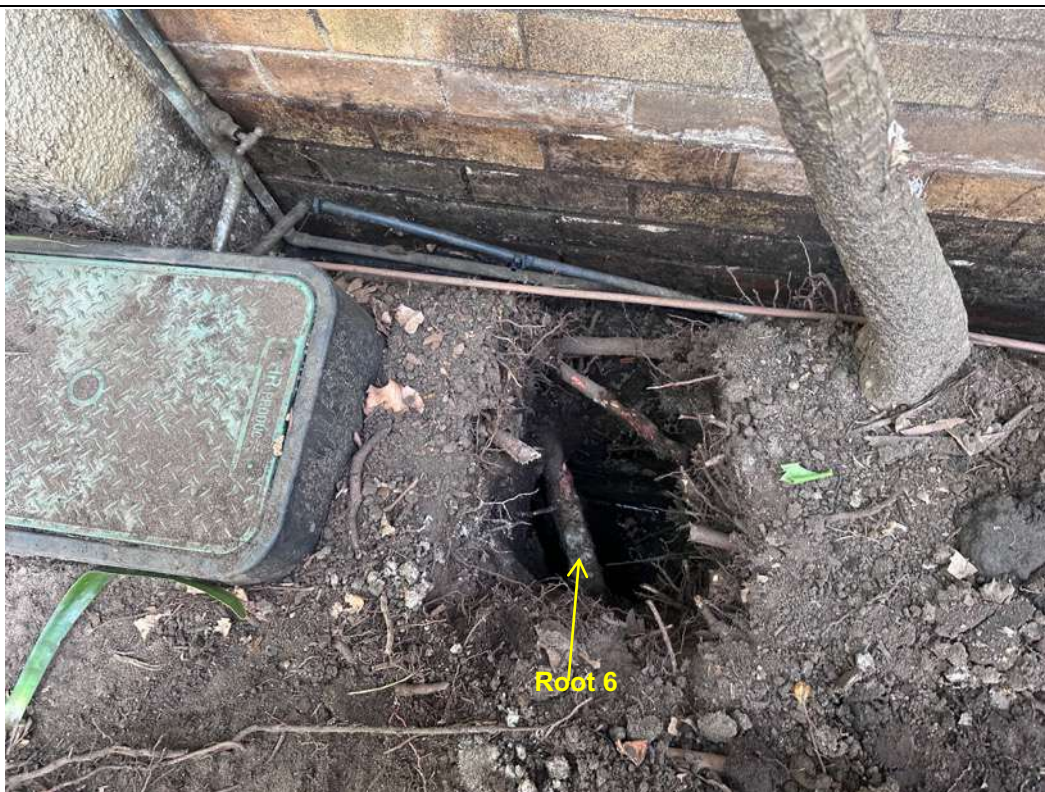
Image 13: Pier 4 and root 6, which extends into trench 2 adjacent to the building footings.
