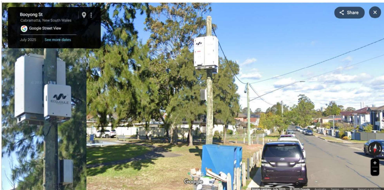
Battery unit, control box and distribution board on pole at Booyong Street, Cabramatta at Bolivia Park. Source: Google Maps Street View.
