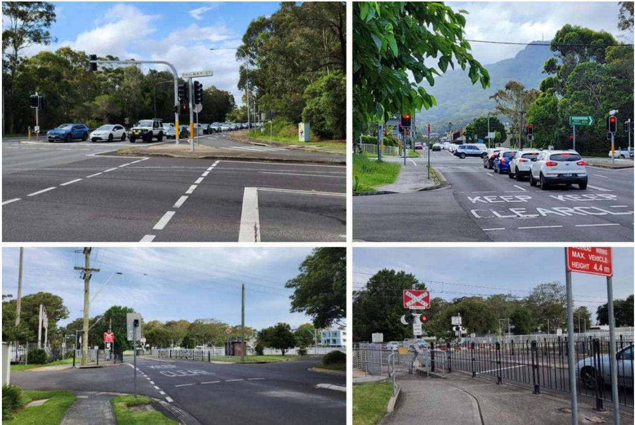
Figure 2.3: Site Visit Photos
