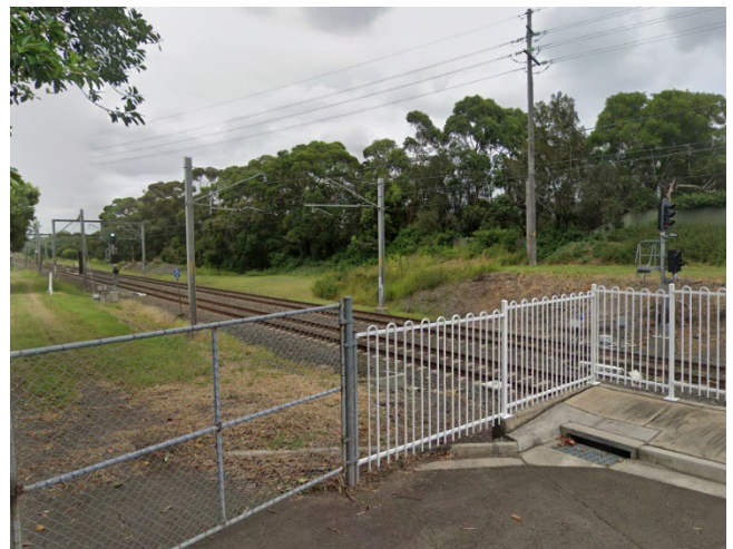
Picture 4 Eastern Boundary – Corrimal Train Station Source: Google Maps 2019
