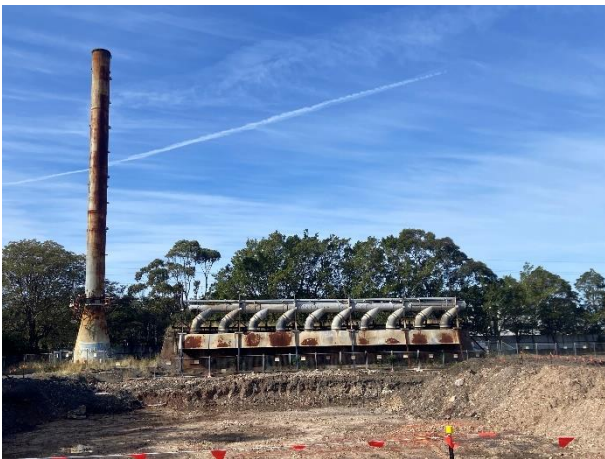
Figure 3 – View east towards the Coke Ovens (north of the subject area).
