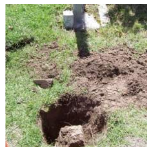
Concrete Block references boundary corner (peg)
