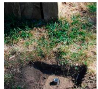
Galvanised Iron Pipe references boundary corner
