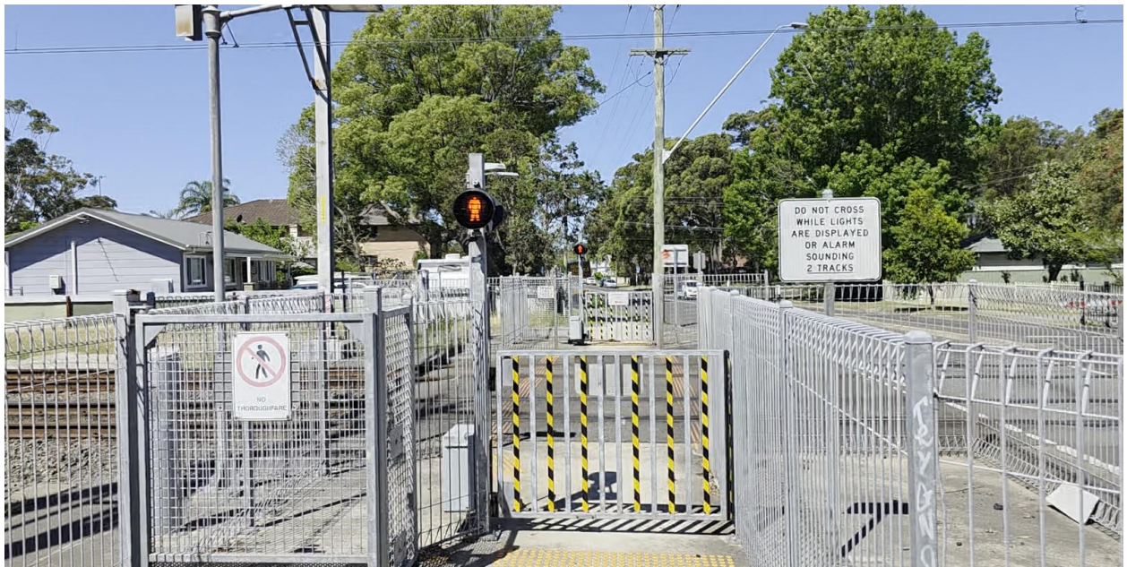
Photo 2 (Photo: Traffic Engineering Centre)
