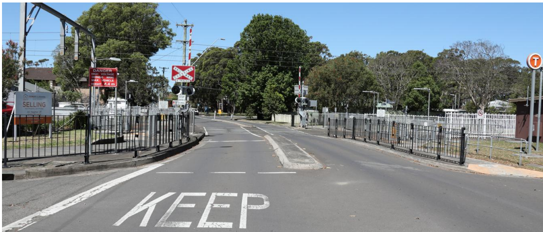
Photo 3.1: Railway Street, on the western approach to the Railway Crossing – in daylight (Photo: Traffic Engineering Centre)
