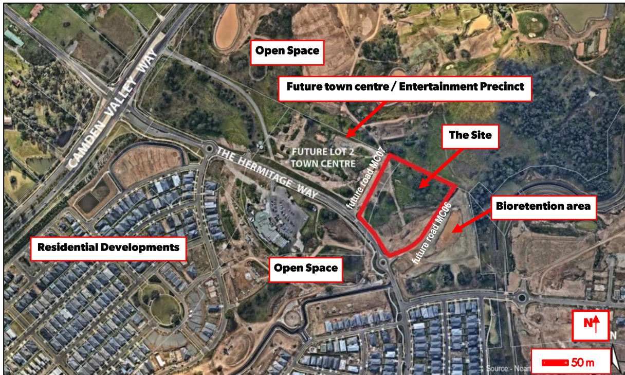
Figure 2 | Aerial image of the site in the context of the surrounding developments (Source: Applicant's EIS)
