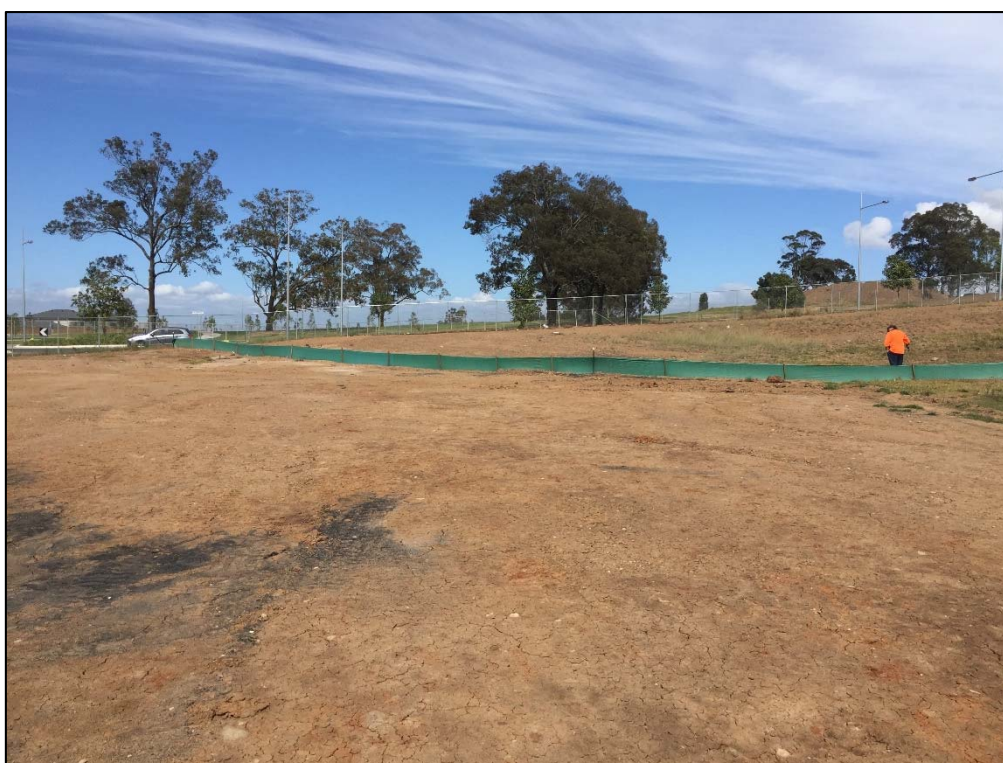
Plate 2: General view across study area, showing silt fencing and grading of ground surface
