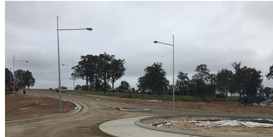
View of the site from the South-East Corner
