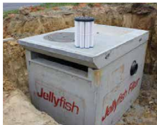
Kerb Inlet Jellyfish Filter is installed in a commercial development
