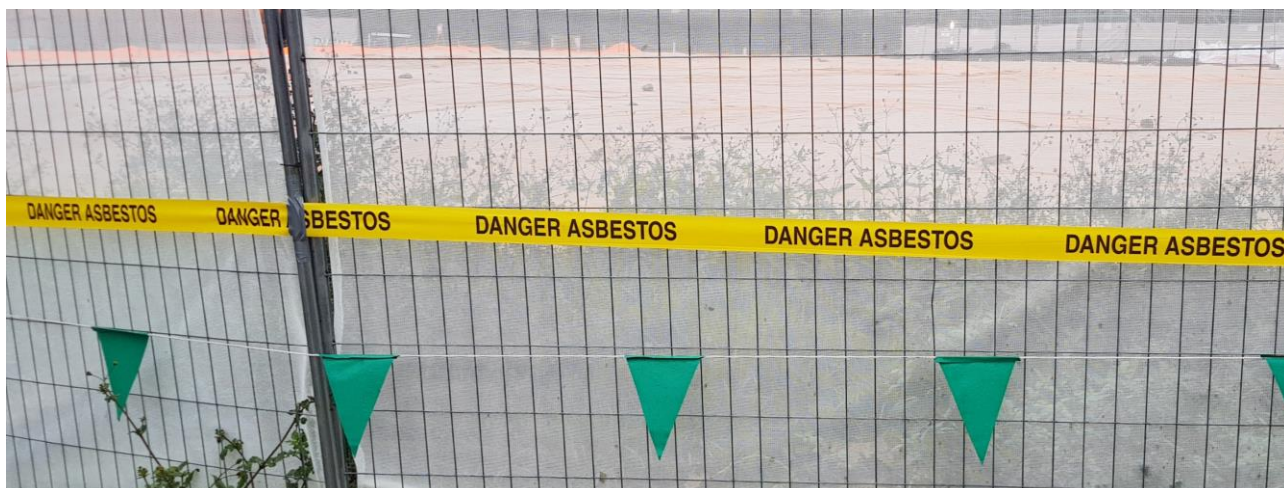
Photo 1: Asbestos barricade and signage.
