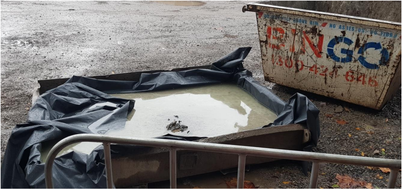
Photo 3: Concrete washout tray.
