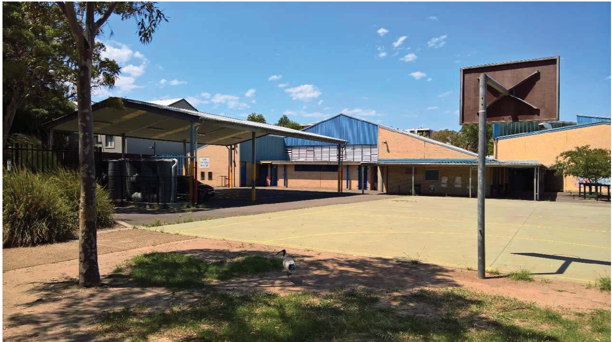
Photograph 6: Basketball court and undercover area within school grounds. School buildings/facilities in view in the background.
